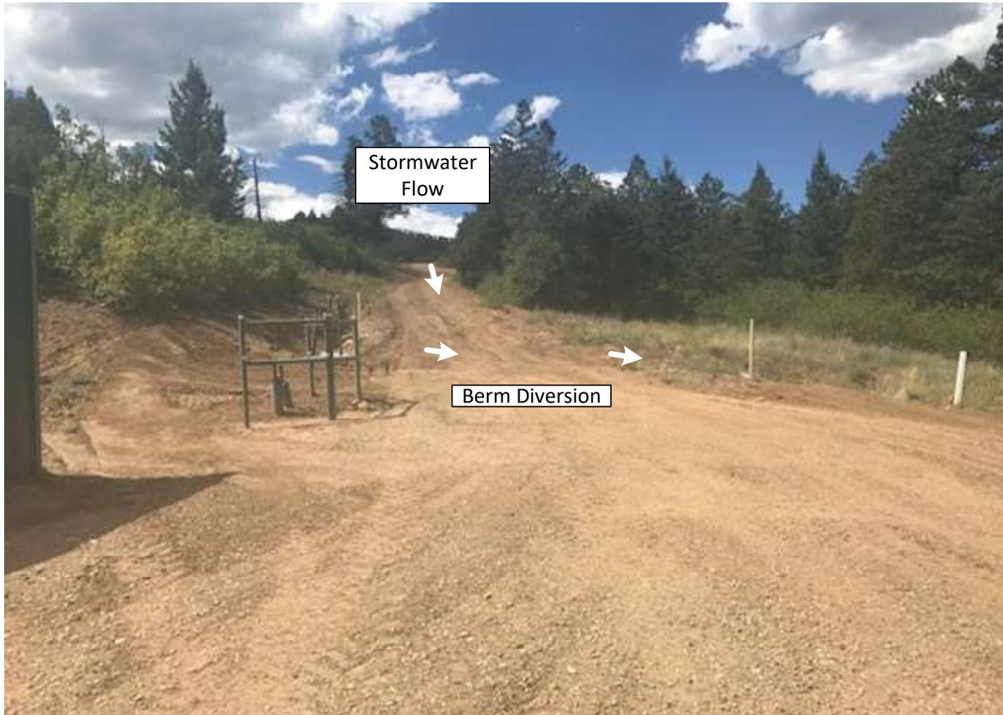
The access road and well pad were regraded to address the rutting and erosion of the access road. Installed a berm diversion across the access road at the entrance to the well pad to direct run on to the culvert outlet, reducing the amount of run on entering the well pad.
