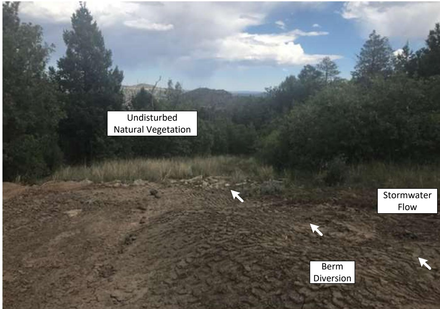
A berm diversion was install on the southern end of the well pad to direct run off to the undisturbed natural vegetation away from the production facilities.
