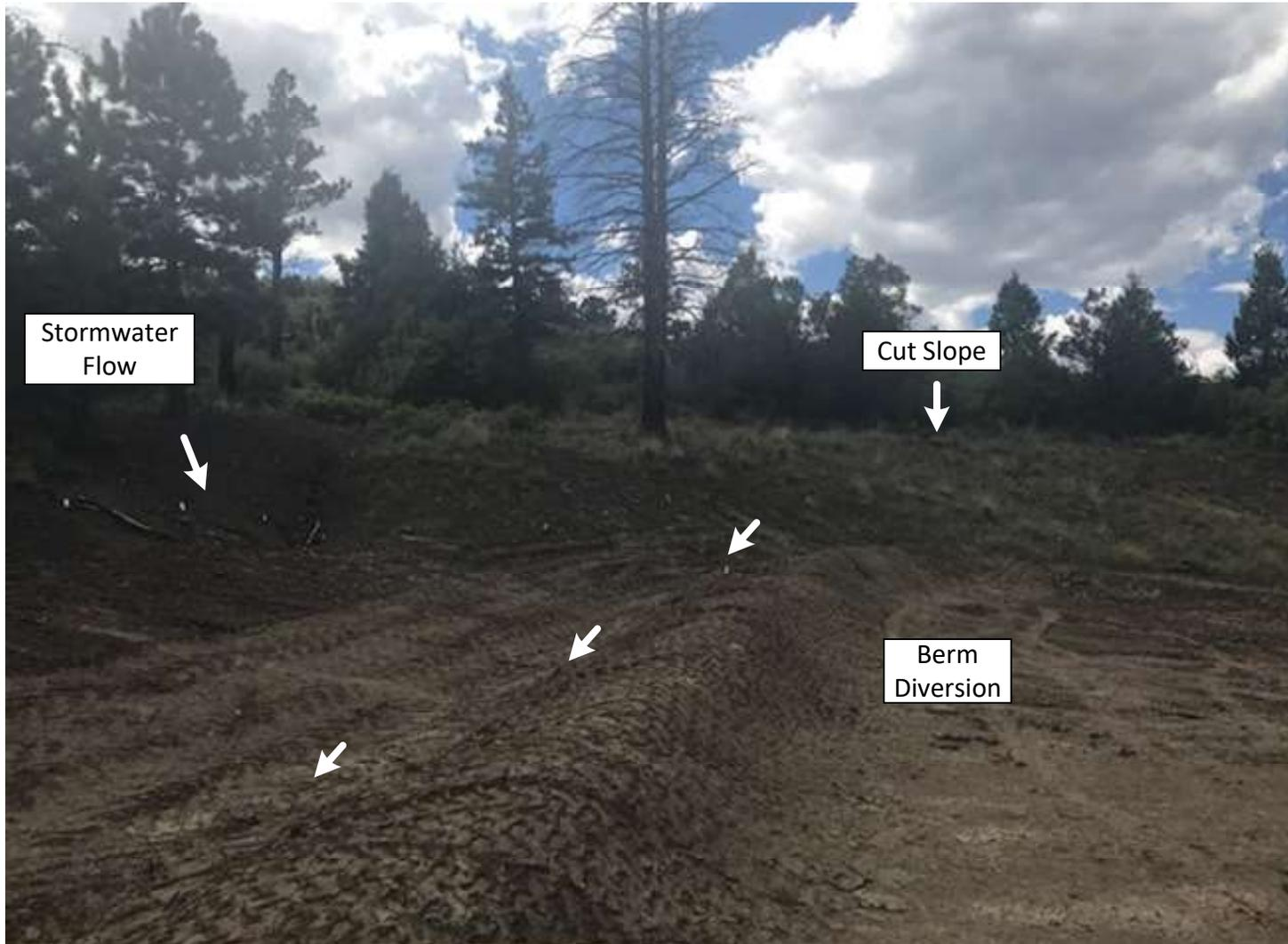
There was a natural drainage that intersected the cut slope, allowing run on to pound on the well pad. A berm diversion was install on the southern end of the well pad to direct run off to the undisturbed natural vegetation.
