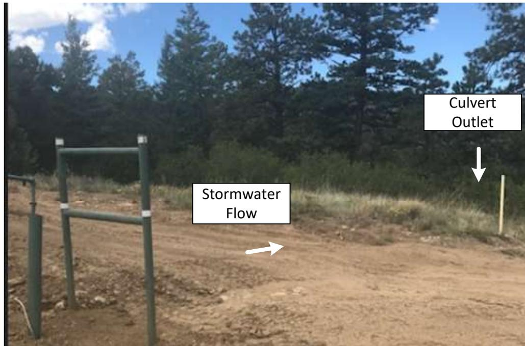
Installed a berm diversion across the access road at the entrance to the well pad to direct run on to the culvert outlet, reducing the amount of run on entering the well pad.
