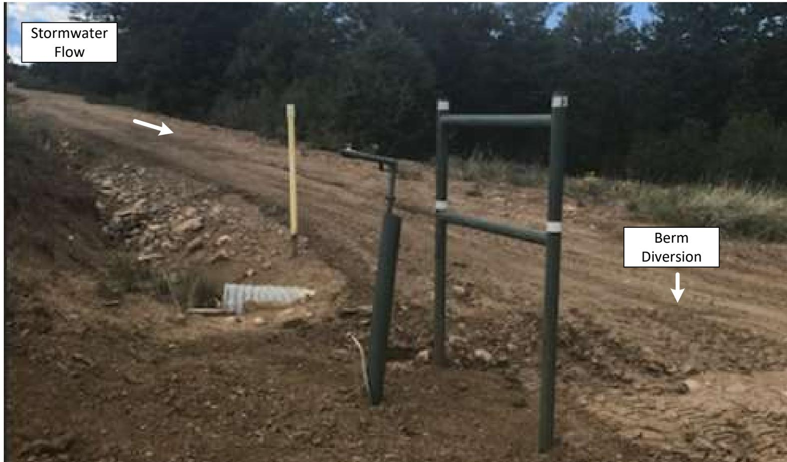
Installed a berm diversion across the access road at the entrance to the well pad to direct run on to the culvert outlet, reducing the amount of run on entering the well pad.
