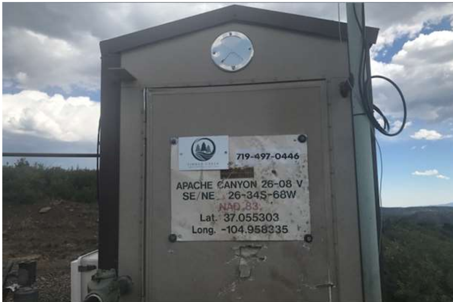
THE LEASE SIGN WAS REATTACHED TO THE SEPARATOR HOUSE USING LARGER WASHERS FOR A MORE SECURE FIT.
