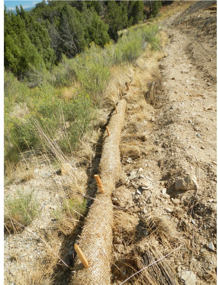
Photo#3: 8/28/18 Wattles have been properly installed
