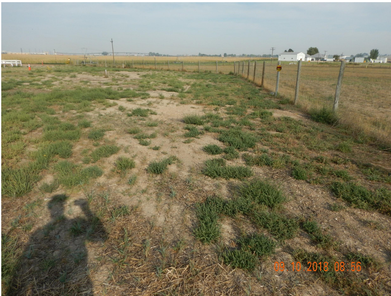
Photo 3. Photo taken from the western tank battery, facing Northwest. See comments under Photo 1. Note: Remediation Project #8315 has not been resolved and remains open until it complies with 900 series rules and regulations. Also, there was little to no germination of grass species throughout portions of the tank battery. Operator should consider taking soil samples to determine soil fertility.
