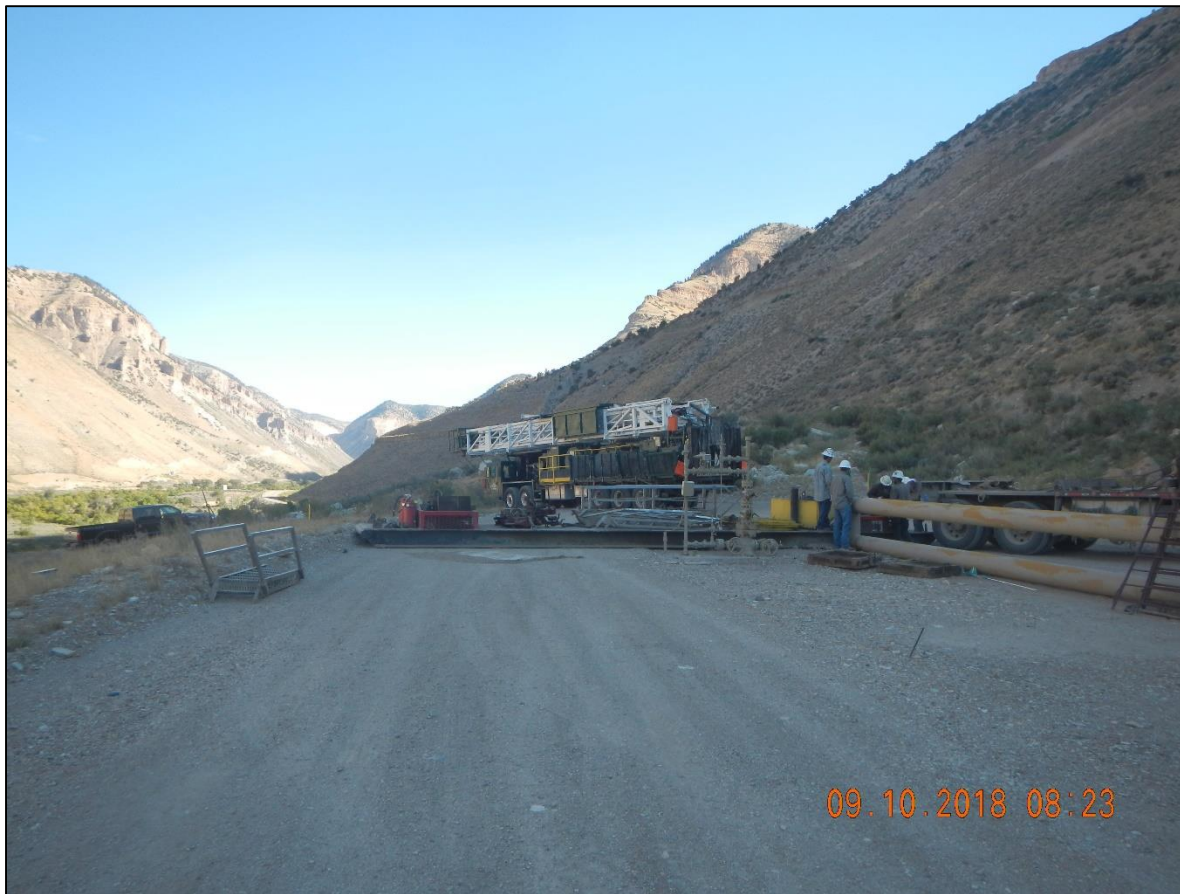
Rigging up work over rig for well abandonment work.
