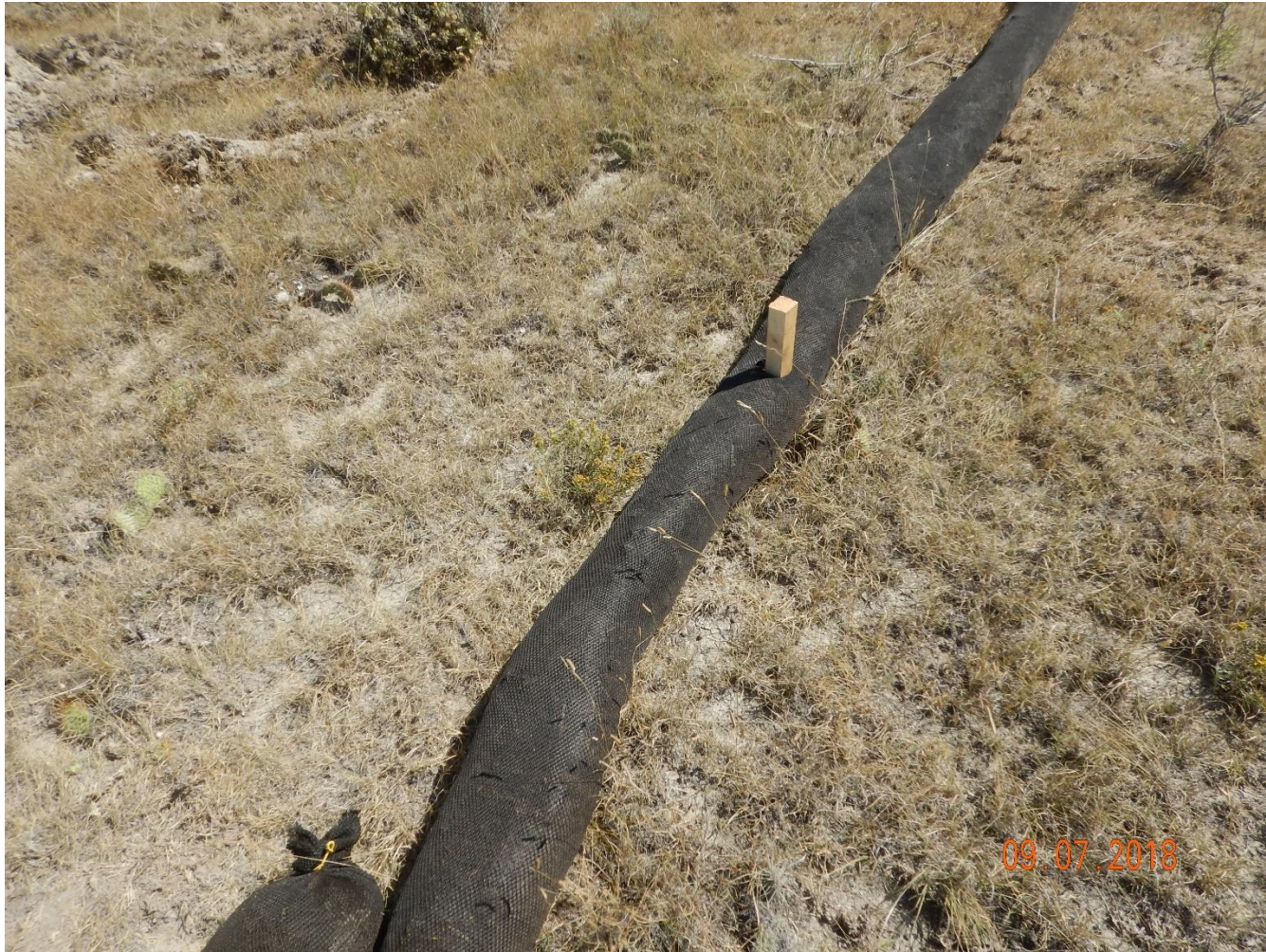
Photo 8: Photo taken from the south end of the location. Photo shows wattle. Wattles have been laid directly upon the soil surface and have not been trenched and back-filled in accordance with good engineering practices; BMP is not in proper functioning condition.
