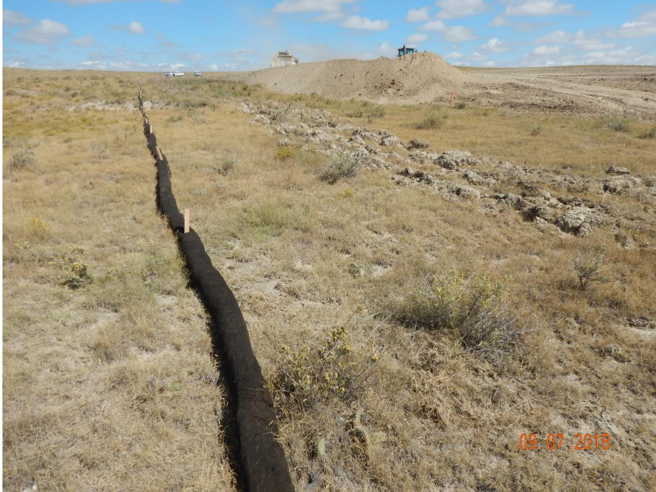
Photo 6: Photo taken from the southwest corner of the location, facing north. Photo shows operator appears to have implemented wattles and surface roughening as stormwater and erosion control BMPs
