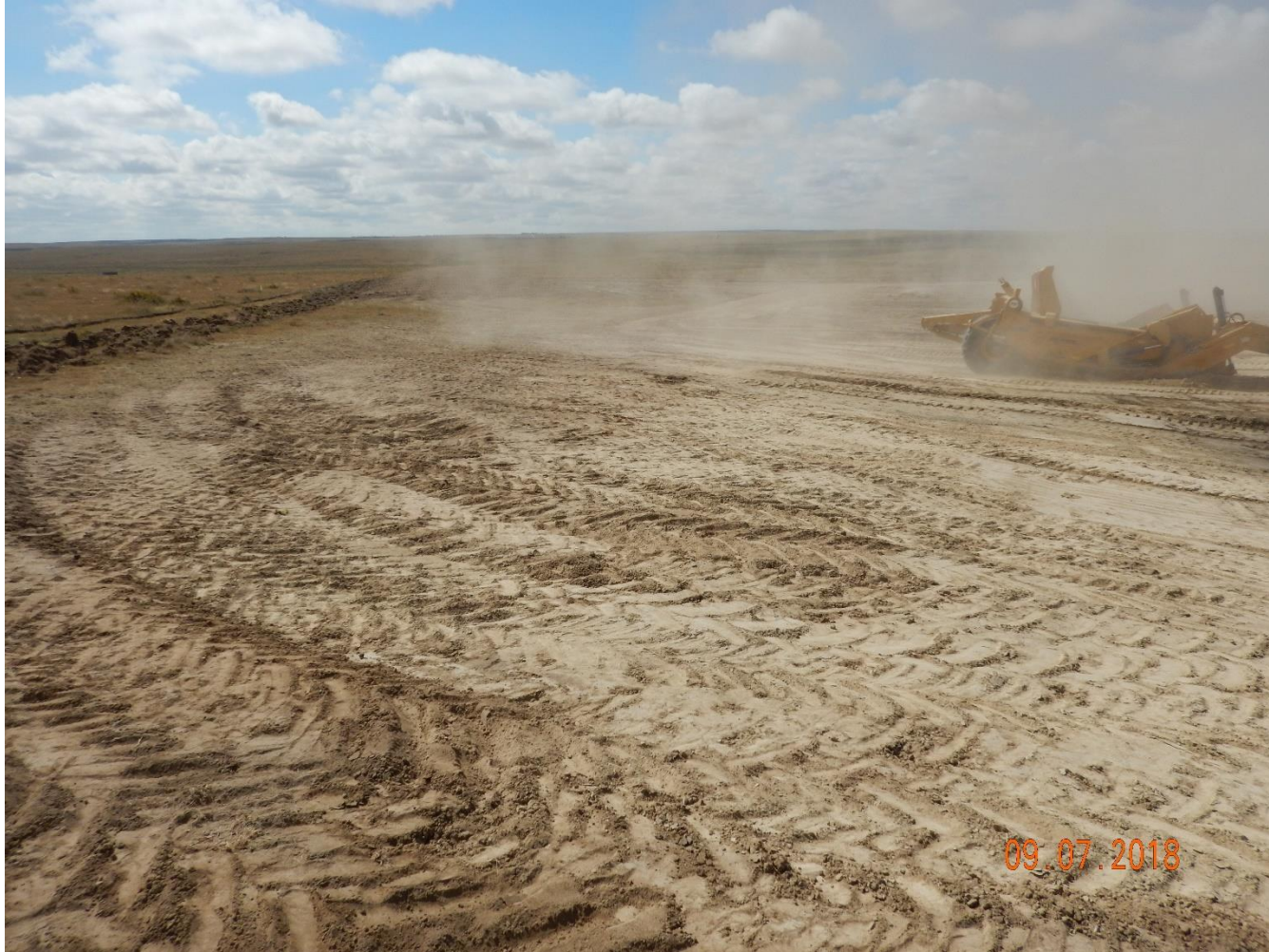
Photo 14: Photo taken from the southeast corner of the pad, facing south. Photo shows contractor scraping soil. Un-salvaged topsoil appears to remain on the pad. Upon contacting contractor operator scraper, inspector was told that topsoil salvage activities have been completed, and that no additional topsoil salvage was planned. Contractor was currently scraping soils to be used as fill material; IT APPEARS AS THOUGH TOPSOIL IS BEING USED AND INCORPORATED AS FILL MATERIAL. SEE PHOTO 10
