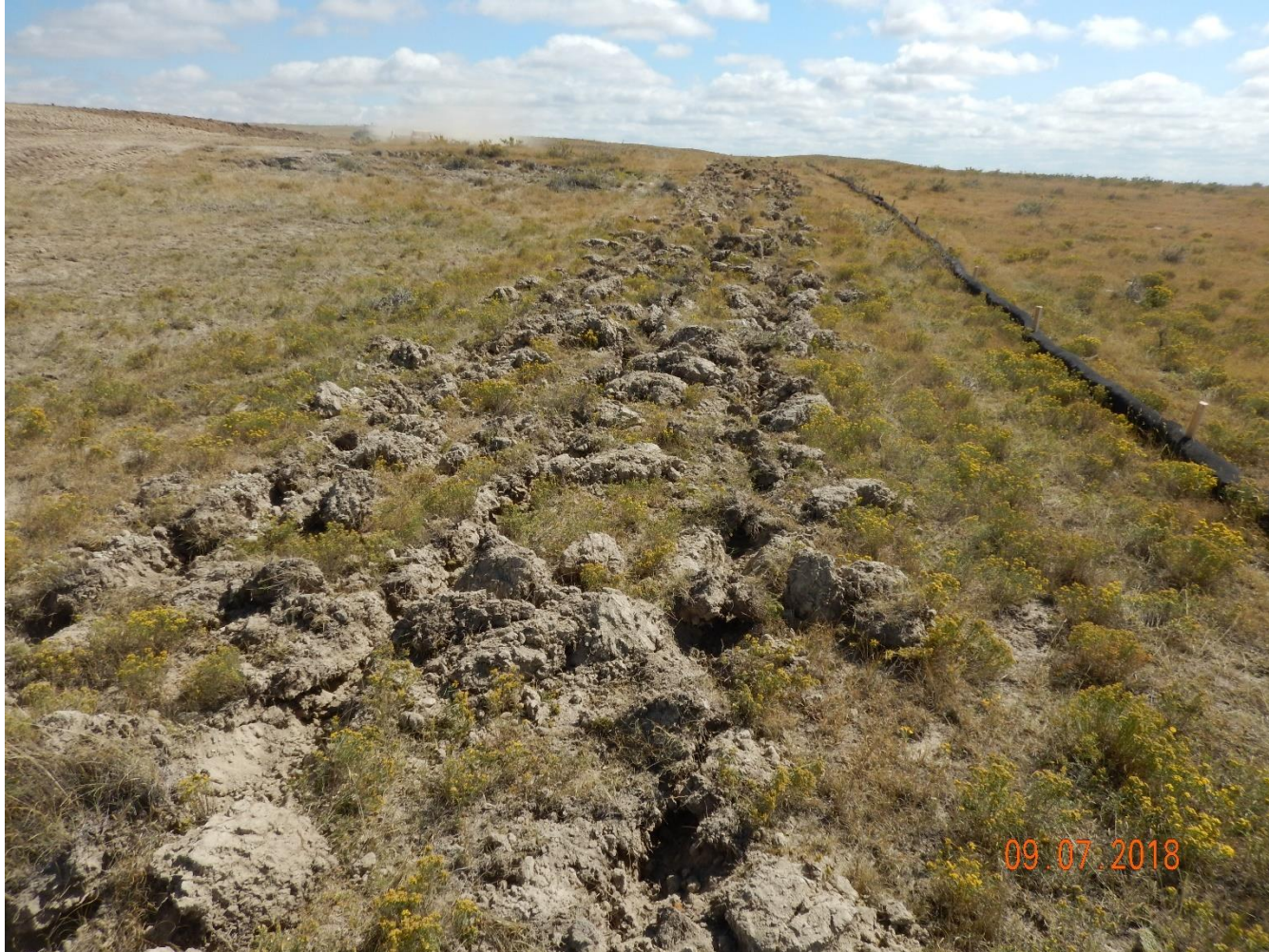
Photo 9: Photo taken from the south end of the location. Photo shows surface roughening BMP along perimeter.
