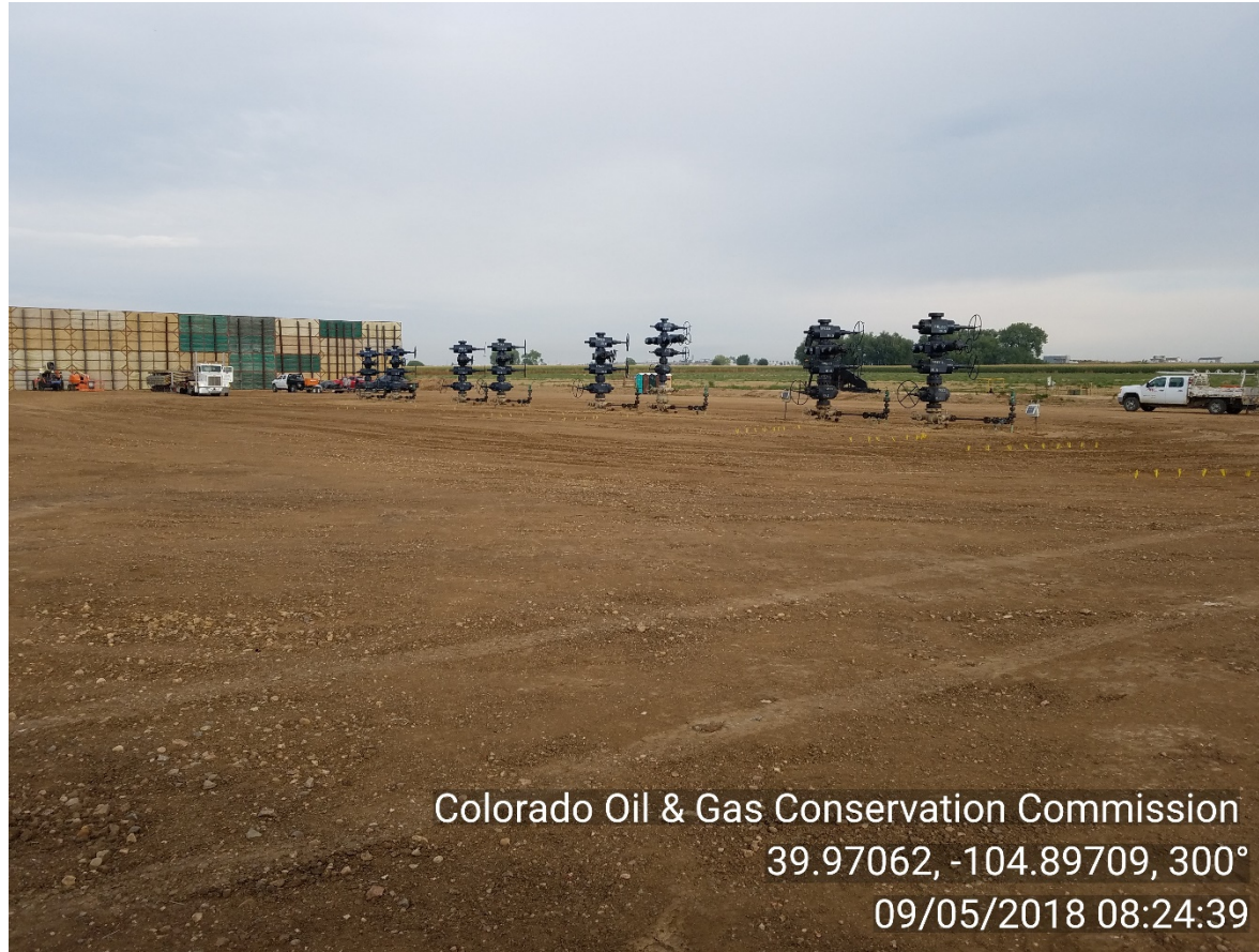
Wellheads & location preparing for flow back.
