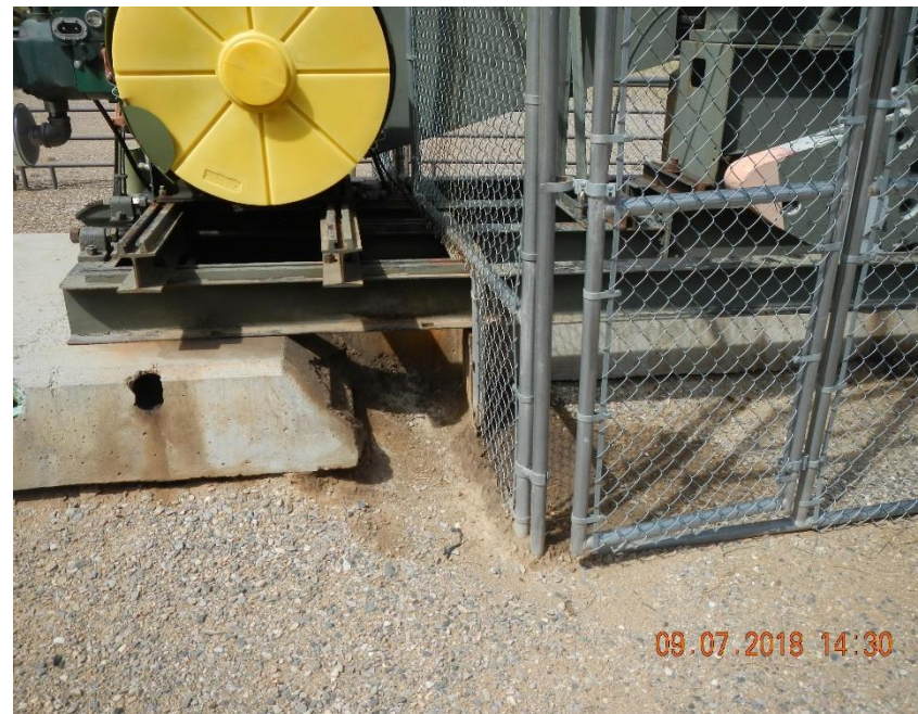
Stained soil near pump jack.
