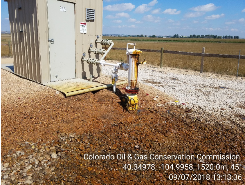
DCP Meter post vehicle strike
