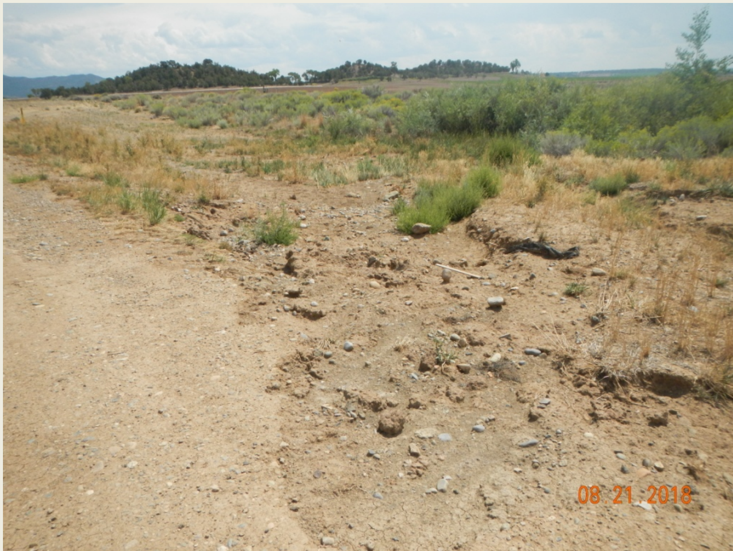
Photo 5. View of erosion and sediment deposition along the access road that needs to be repaired, facing southeastward.
