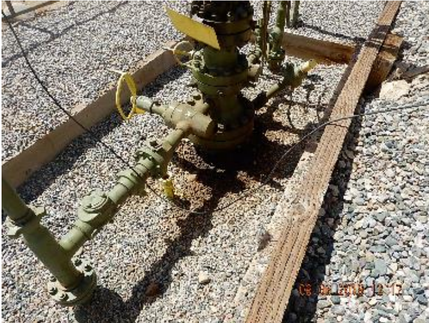
Photo 3: Impacted soil and gravel around base of C #1 wellhead.
