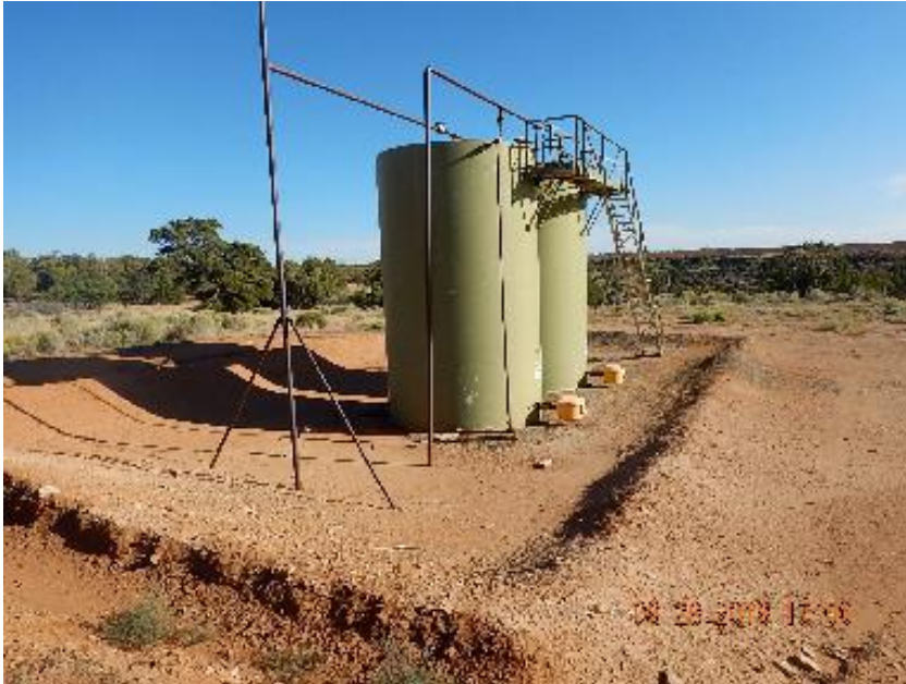
Photo 7: Production tanks and flow line to tanks. Flowline at separator appear to of been abandoned.
