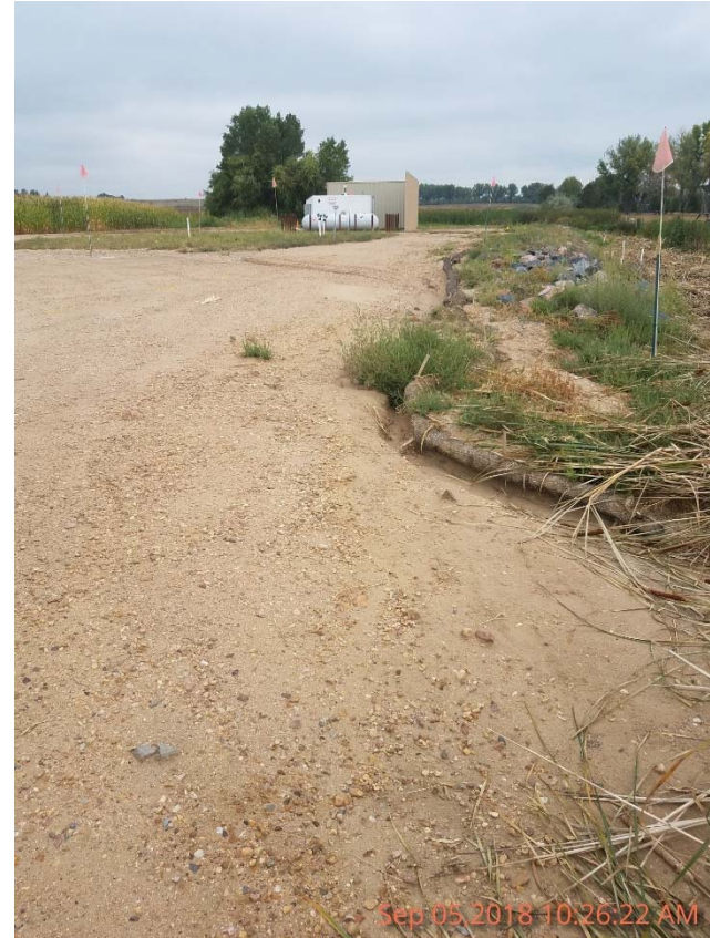
Photo 4 – Rill forming from stormwater runoff. Stormwater controls require maintenance.
