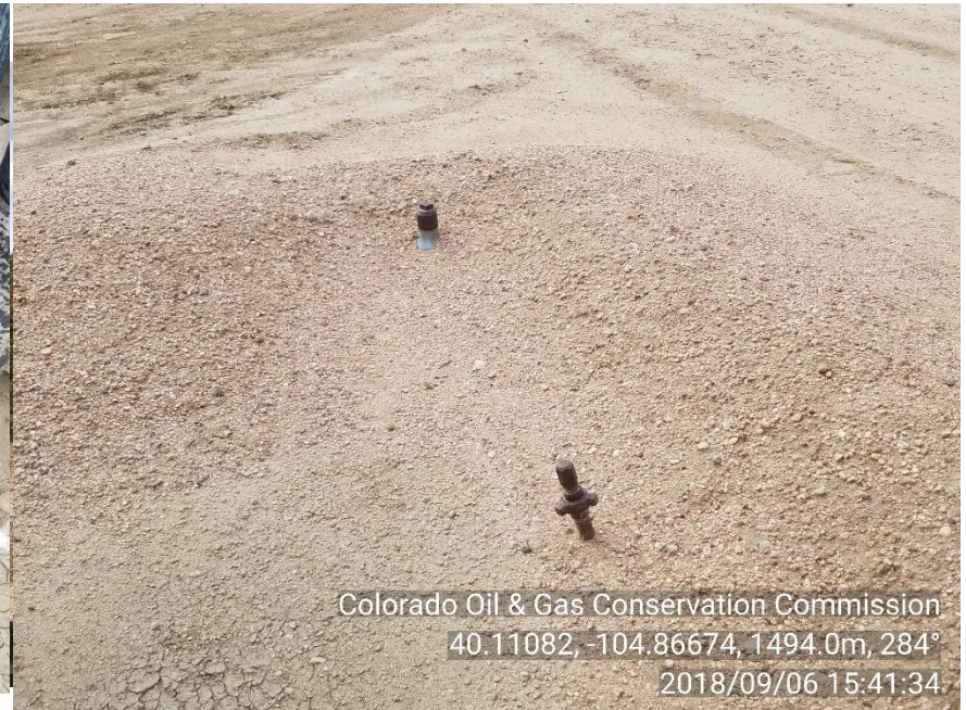
Photo 8. Unmarked riser
