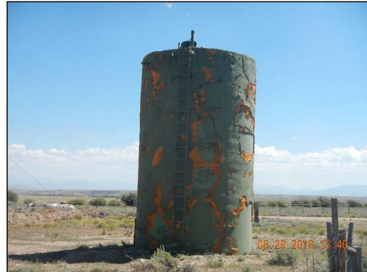
**Photo 4. Tank with no berm and no label.**
