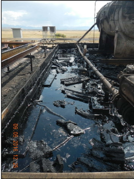
Photo 9. Close-up overview of fluids and debris present in berm of separator 1 of 3.
