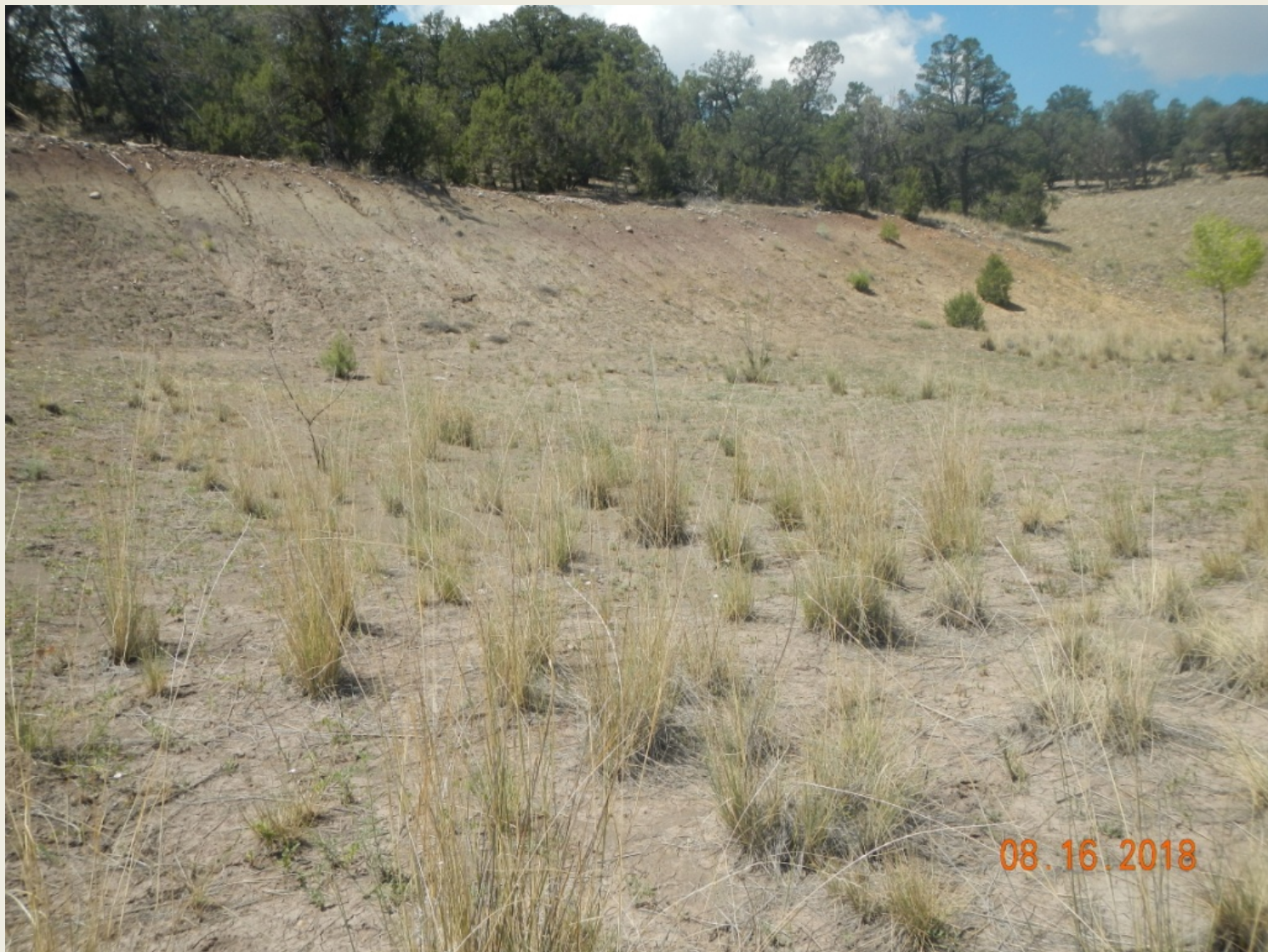
Photo 7. View of the southern and southwestern cut-slope from the southern edge facing westward. Erosion is occurring in this portion of the cut-slope near the top where vegetation is not established.
