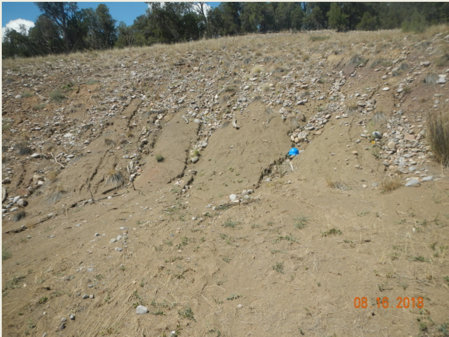
Photo 5. View of erosional channels and sediment deposition within the northwestern cut-slope.
