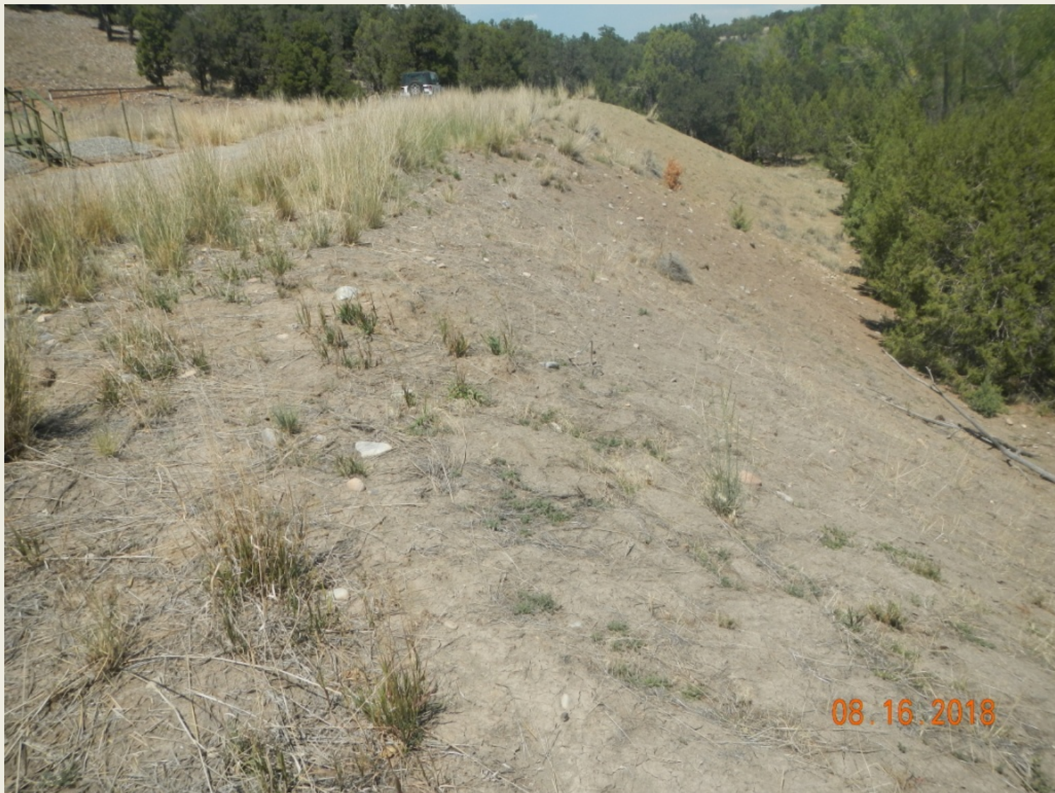
Photo 3. View of the eastern portion of the project area from the southeastern corner facing northward. Revegetation is sparse on the fill slope. Many grasses appear to be dried out.
