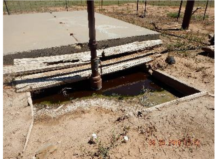
Photo 4: Wellhead cellar with standing fluids. Current inspection.
