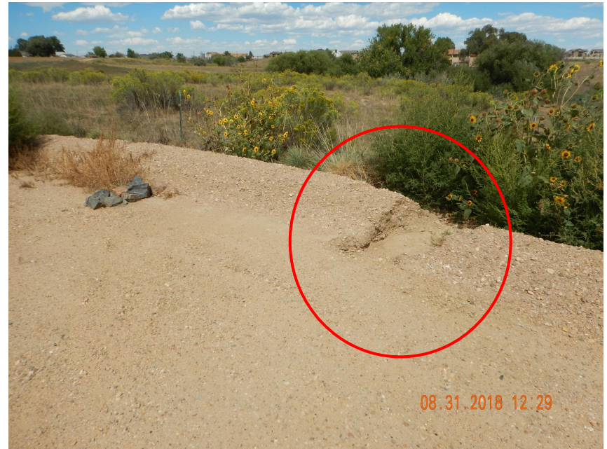
Photo 2. Photo taken of the northern battery location, facing North. Berm BMP in need of repair. Sediment discharge was observed off location.
