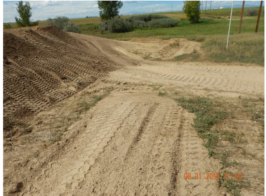
Photo 2. Photo taken from the northwestern perimeter of the location, facing West. Photo illustrates where a culvert is needed in conjunction with the ditch and berm BMP.
