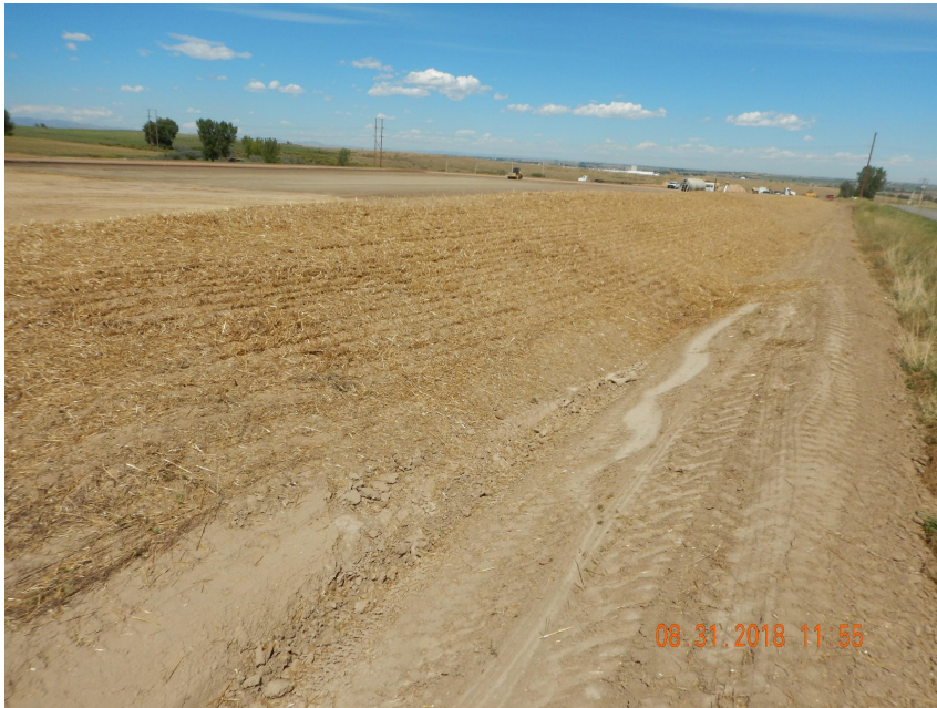
Photo 5. Photo taken from the southeastern perimeter of the location, facing North. Topsoil has been salvaged and stored along the western and eastern perimeter of the location. Topsoil has been seeded, straw mulched and crimped.
