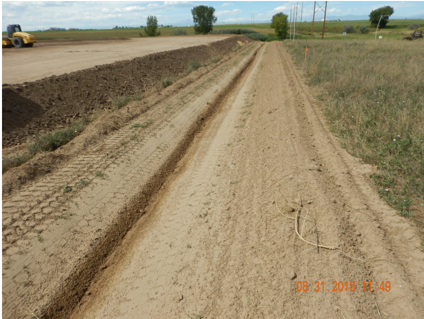
Photo 1. Photo taken from the northeast perimeter of the location, facing West. Ditch and berm BMP has been installed around the entire perimeter of the location. Culverts are needed and were staged on location.
