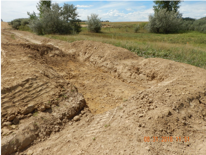
Photo 3. Photo taken from the northwest perimeter of the location, facing Southwest. Sediment trap is IN-PROCESS of being constructed. Sediment trap lacks both inlet and outlet protection devices.
