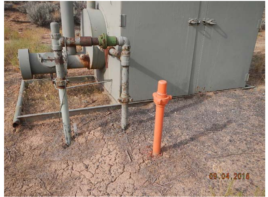
Photo 2. Marked and bull-plugged riser
