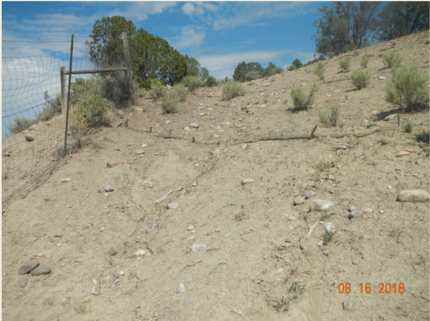
Photo 7. View of erosion occurring in the northwestern corner of the project area. Wattles do not appear to be functioning and are not sufficient stormwater controls for the slope.
