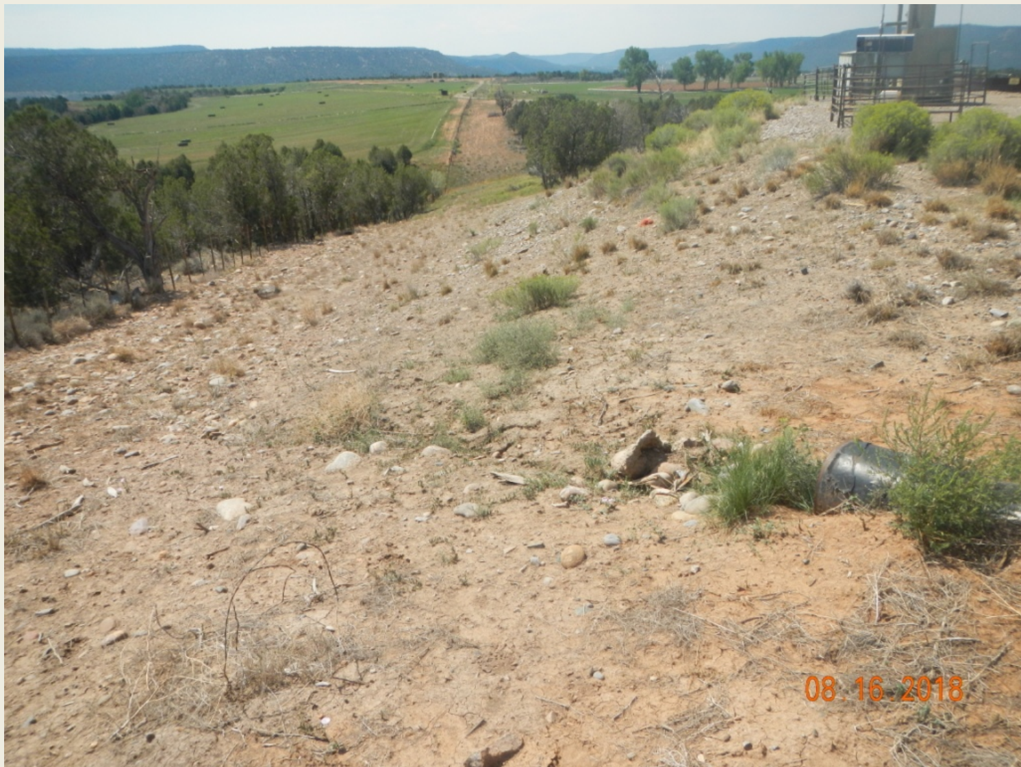
Photo 4. View of wire debris and erosional channel forming at the culvert outlet in the northeastern portion of the project area.
