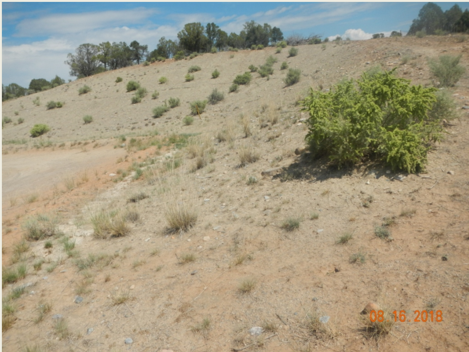
Photo 5. View of the northern and northeastern cut-slopes from the northeastern edge facing northwestward. Vegetation is sparse on the cut-slope and erosion is occurring in several areas.
