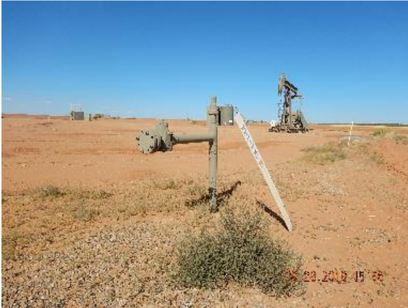
Photo 3: Unused 3" steel riser in SW corner of location.
