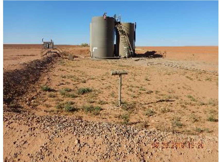
Photo 4: Unused 2" steel riser in SW corner of tank battery.
