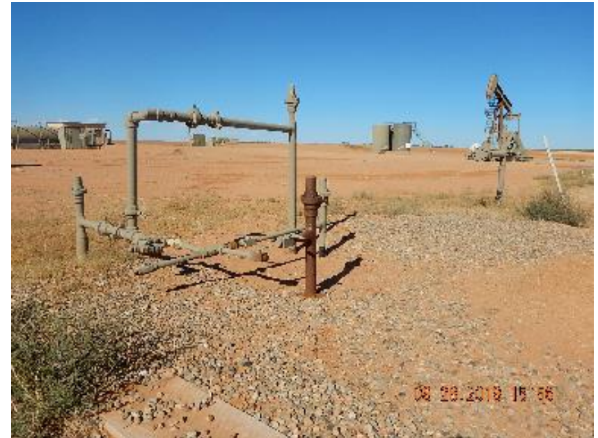
Photo 2: Unused 2" steel riser in SW corner of location.
