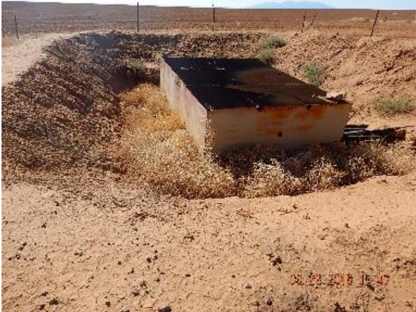
Photo 5: Dried weed debris trapped inside pit around blow down tank.
