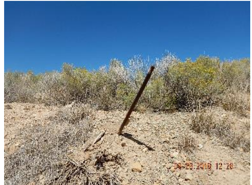
Photo 2: Unused 2" steel riser on S fill slope.
