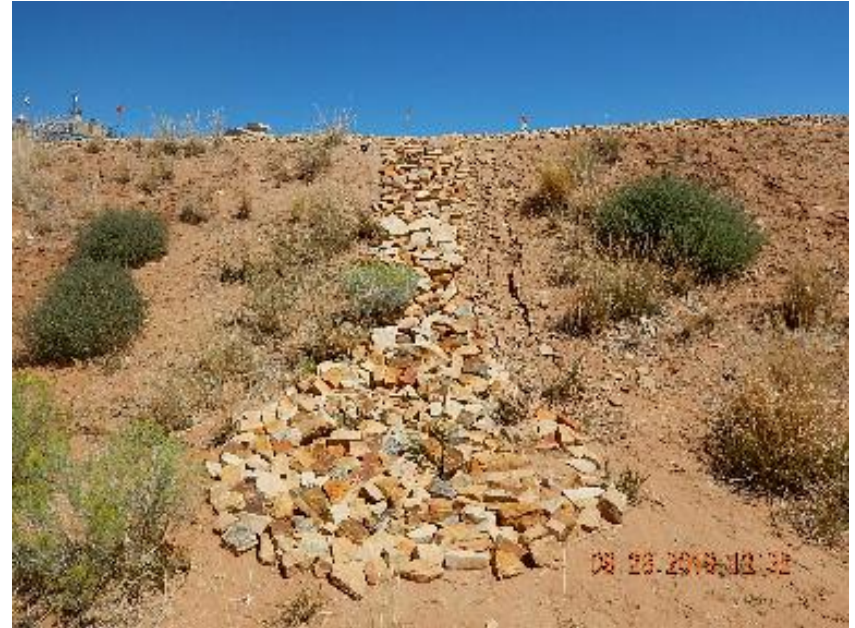
Photo 4: Noted rilling down the edge of rock BMP on W fill slope.
