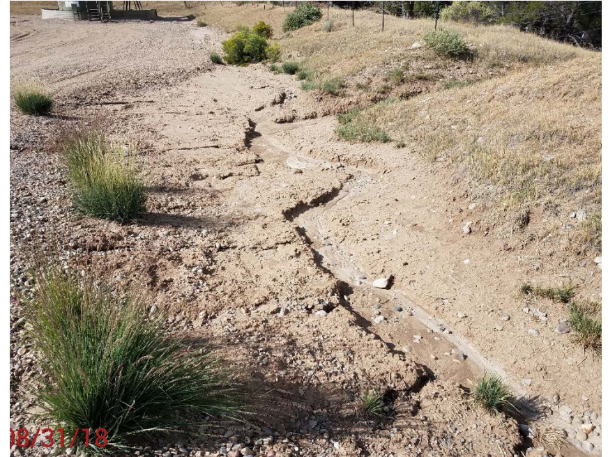
Location Photo #2, soil movement off of location.
