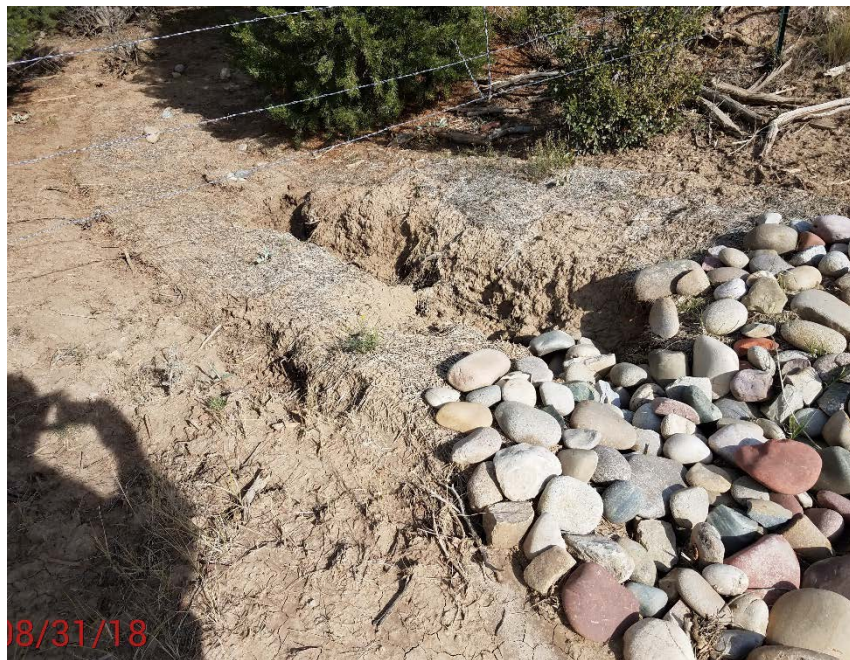
Location Photo #7, Rilling below rip rap in sediment pond.
