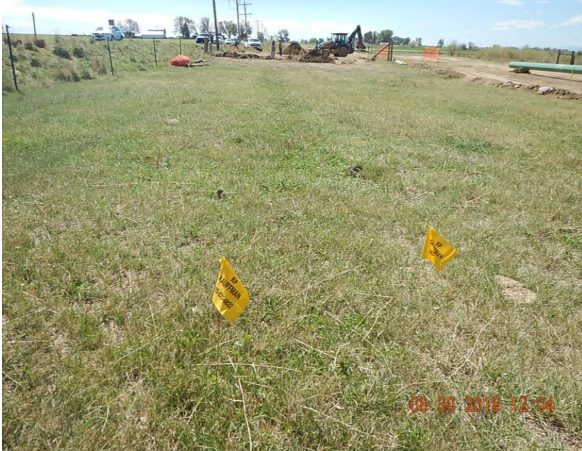
View of excavation area and line locates (pin flags) marking the KPK flowlines routed N-S to the area of release. View to South.
