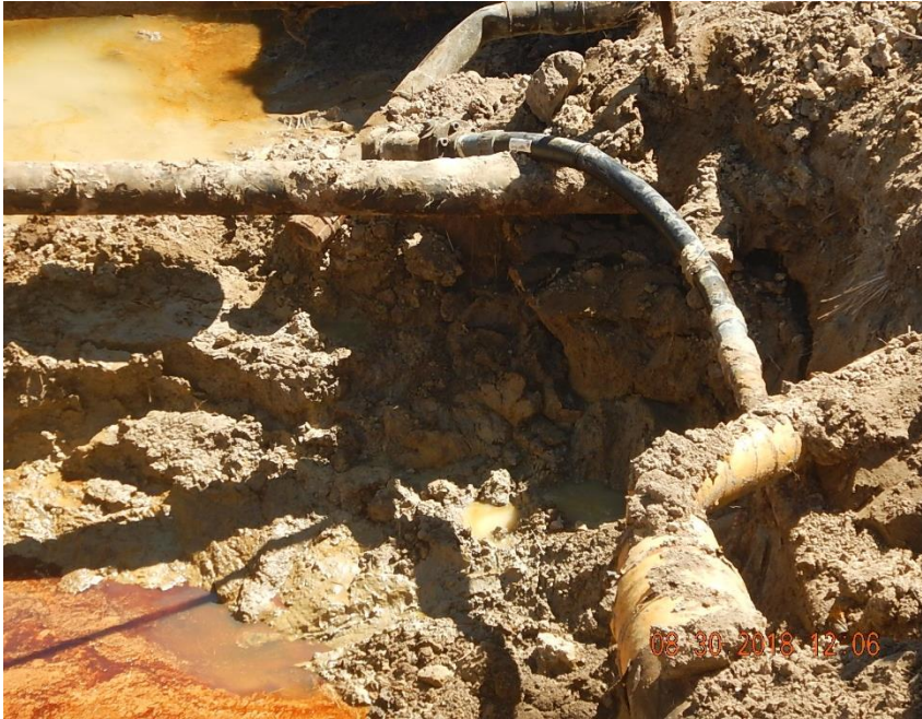
Close up view of flowlines exposed in excavation; The release appears to be a result of the kink observed on the 3" poly flowline although more than one integrity issue may exist.
