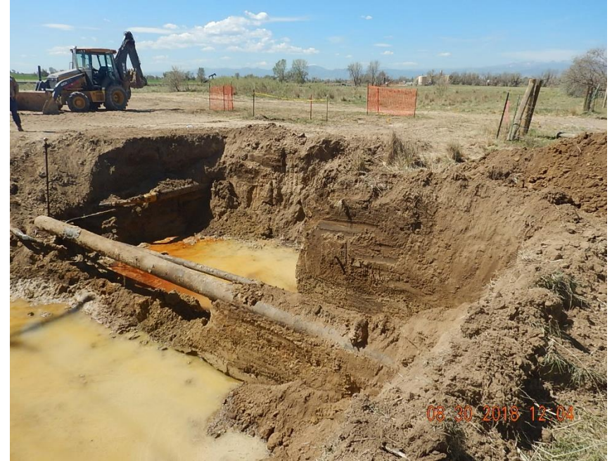
View into excavation showing flowlines exposed; Oil sheen apparent on standing groundwater in the excavation.
