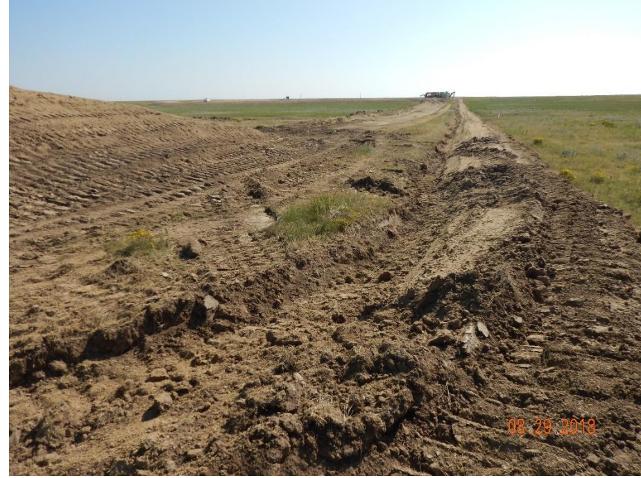
Photo 24: Photo taken from the southwest corner of the location, facing east. Photo shows the stormwater ditch along the perimeter of the location.
