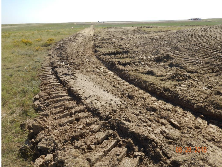
Photo 26: Photo taken from the northwest corner of the locaiton, facing east. Photo shows the stormwater ditch along the perimeter of the location.
