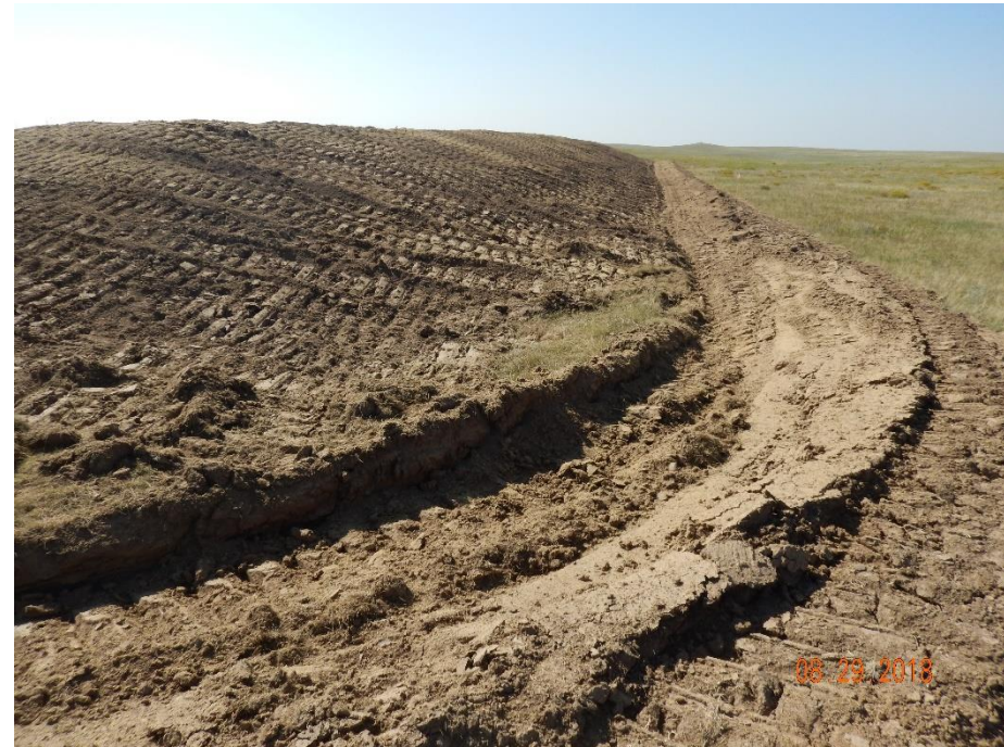
Photo 27: Photo taken from the northwest corner of the locaiton, facing south. Photo shows the stormwater ditch along the perimeter of the location.
