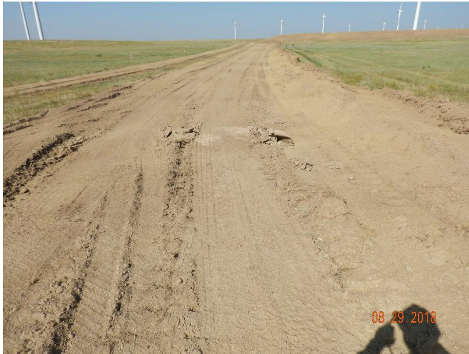
Photo 21: Photo taken from the southwest end of the pad, facing west. Photo shows area where equipment traveled from the pad to the topsoil pile on the west end of the location. Operator appears to have applied a tackifier to these areas for soil stabilization.
