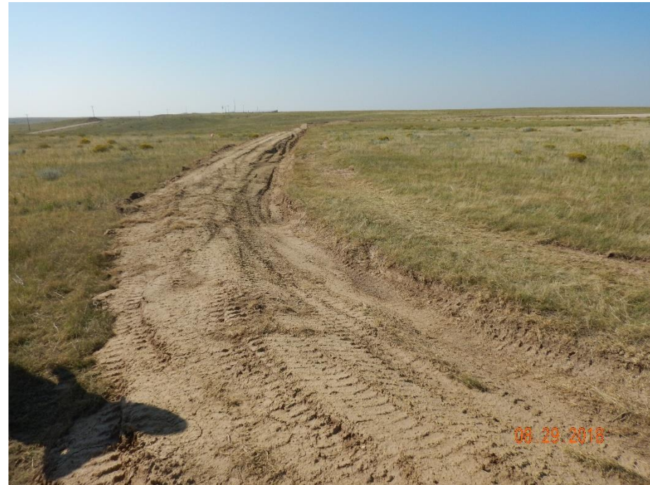
Photo 10: Photo taken from northeast end of the location, facing south. Photo shows the stormwater ditch along the perimeter of the location.
