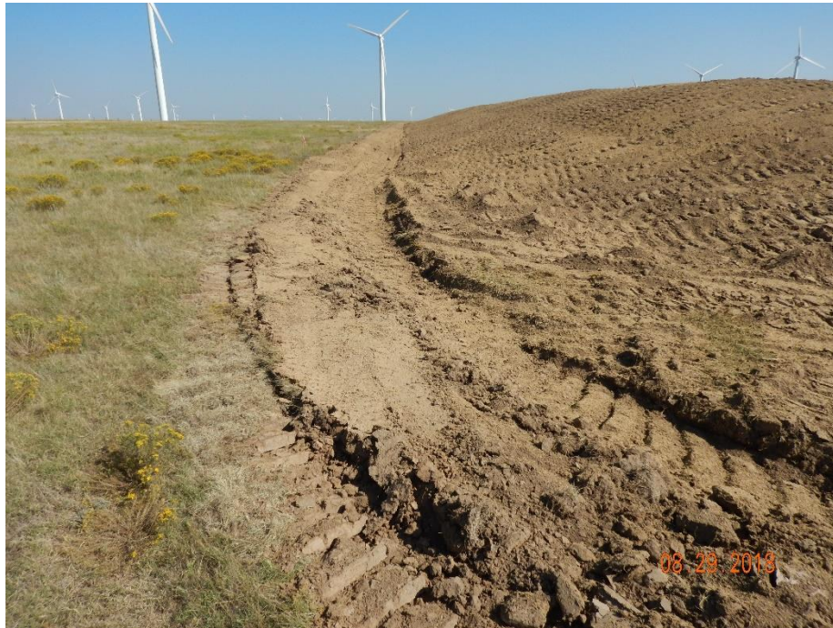
Photo 25: Photo taken from the southwest corner of the location, facing north. Photo shows the stormwater ditch along the perimeter of the location.
