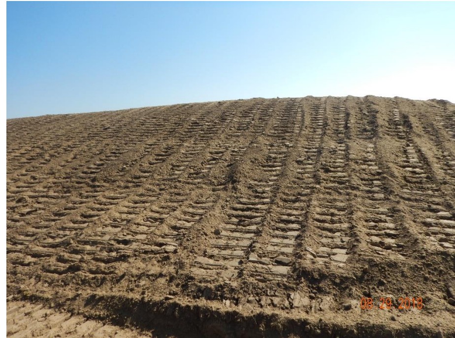
Photo 26: Photo taken from the west end of the location, facing northeast. Photo shows slopes of the topsoil stockpile have been tracked and a tackifier applied for stabilization.
