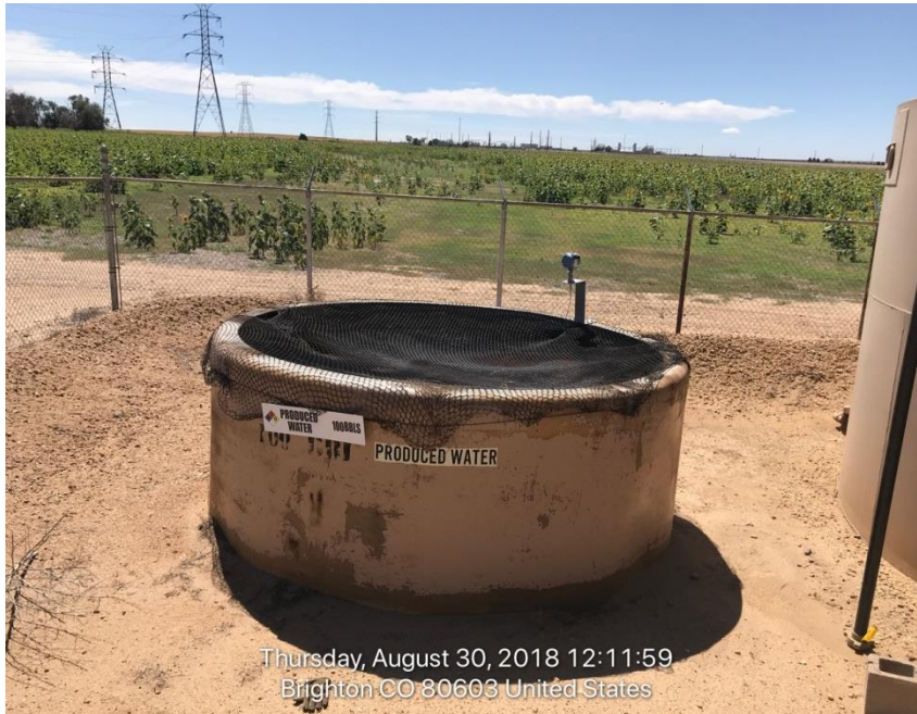
Photo#5 Corrective Action/Netting on open tank inadequate. Holes that wildlife can get into.
