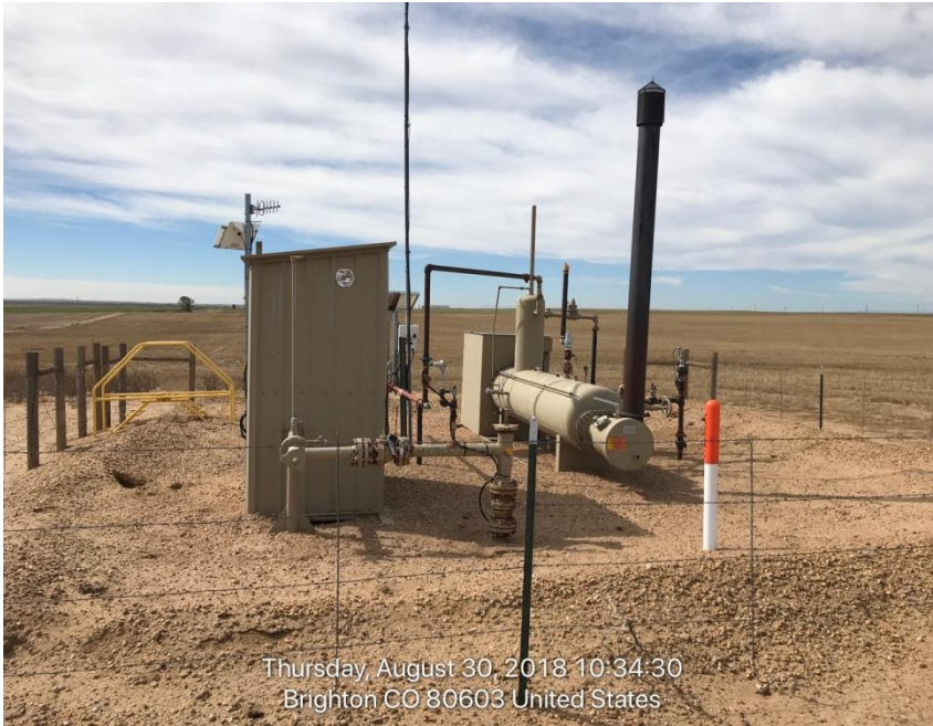
Photo#3 Separator and Gas Meter
