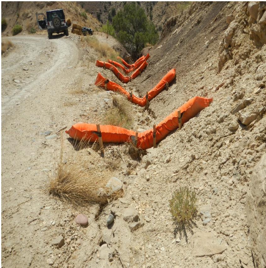
Photo#5: BMPs along Access Road needing maintenance or repair.
