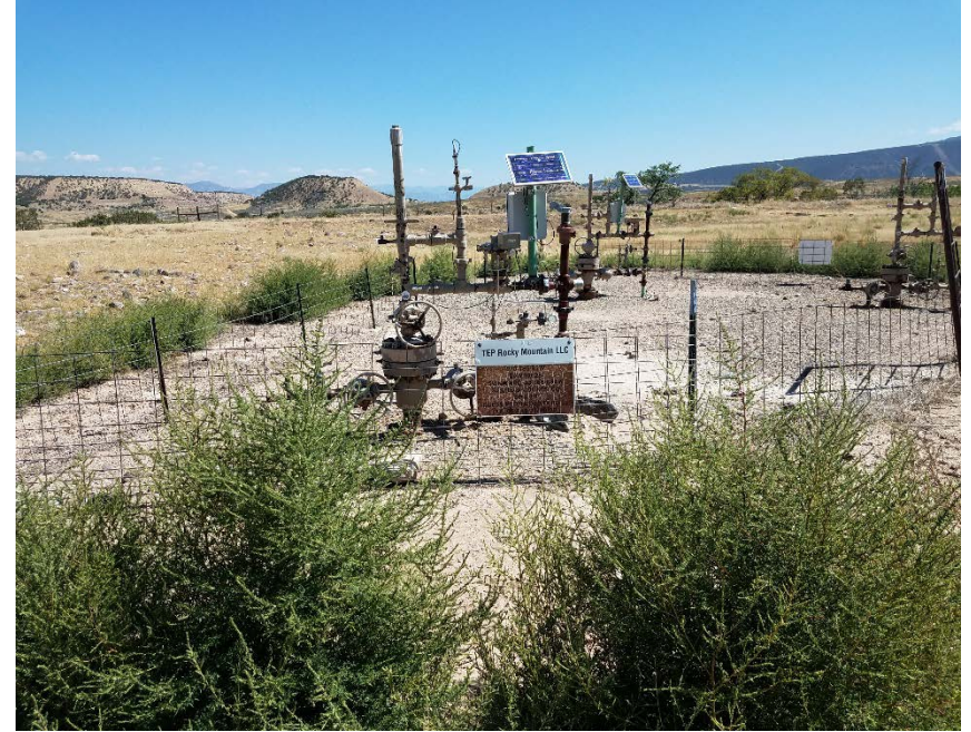
Location Photo #6, weeds around well head, and non legible sign.
