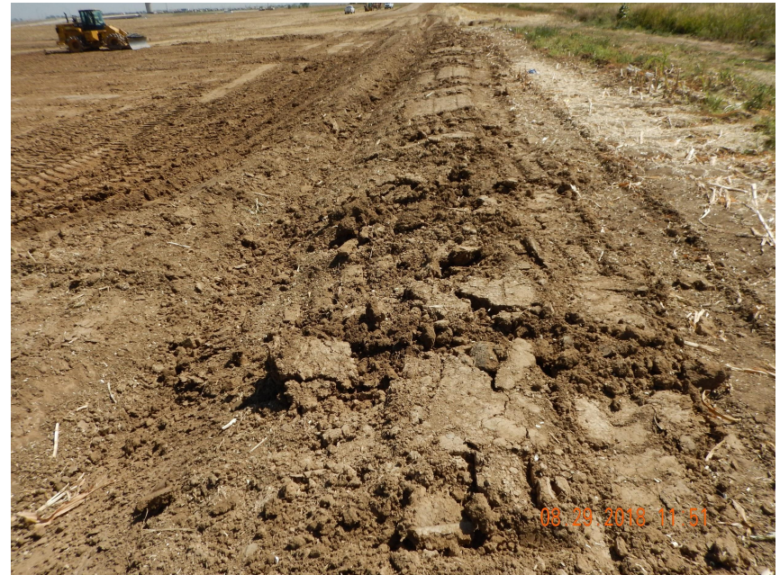
Photo 4. Photo taken from the southern perimeter of the location, facing East. Equipment traffic has damaged a portion of the stormwater BMP. BMPs shall be in proper functioning condition and shall be repaired.
