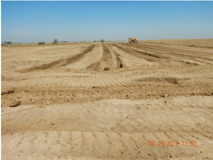
Photo 5. Photo taken from the southern perimeter of the location, facing North. Photo illustrates topsoil salvage operations are underway.
