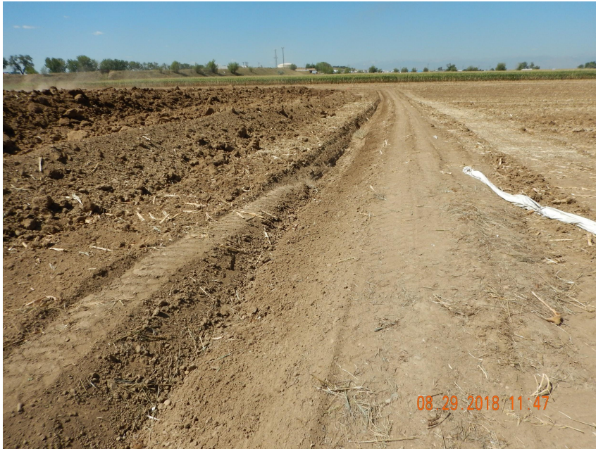
Photo 1. Photo taken from the northern perimeter of the location, facing West. Ditch and berm BMP has been installed along the entire perimeter of the location.
