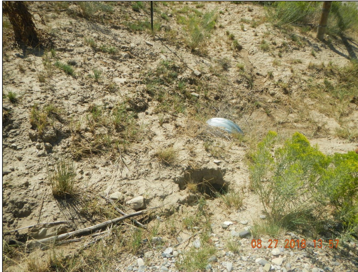
Wash away around culvert.
