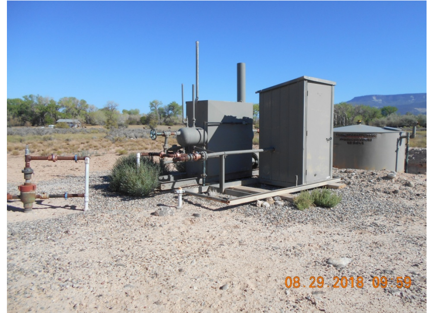
Meter housing, Separator and Tank
