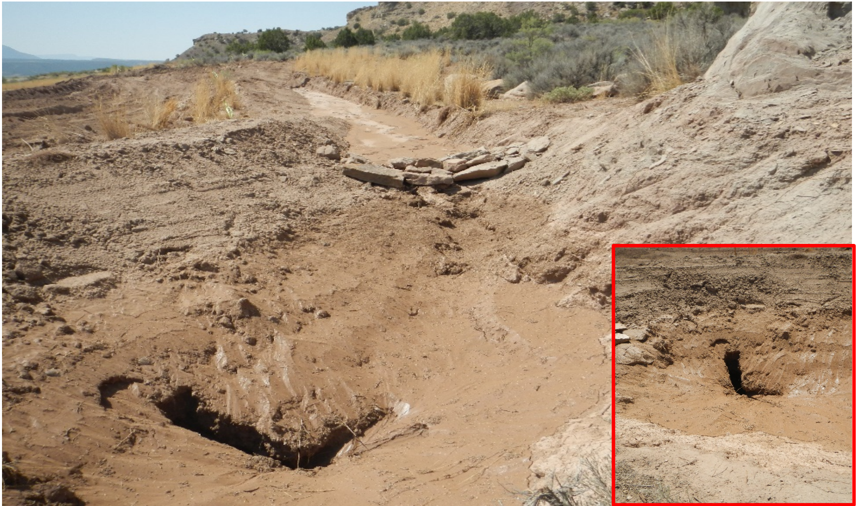
Photo#3: One BMP failure was noted on Northwest corner of Site.
