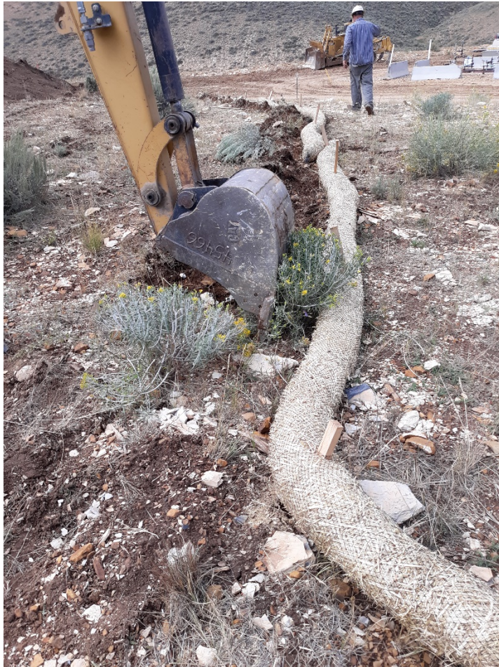
Photo#4: BMPs being installed around Location Perimeter
