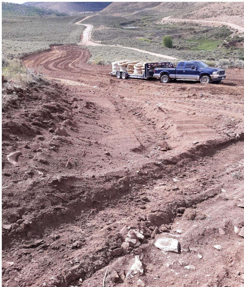
Photo#3: Wattles (or other BMP) not yet installed along Fill side of Access road.
