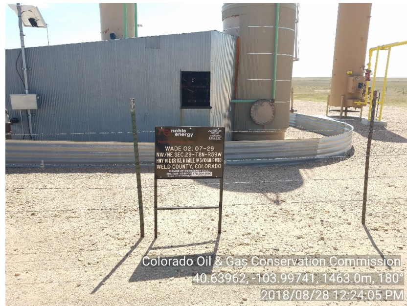
Photo #4 Wade 2-29 Battery View 2
