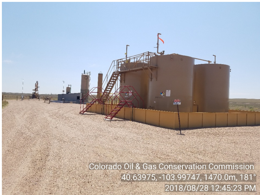
Photo #3 Wade 2-29 Battery View 1
