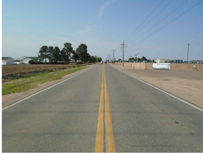
VIEW NORTH (COUNTY ROAD 27)
