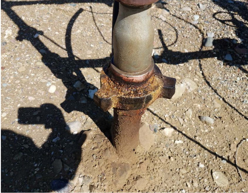
Location Photo #6, leaking fitting at wellhead
