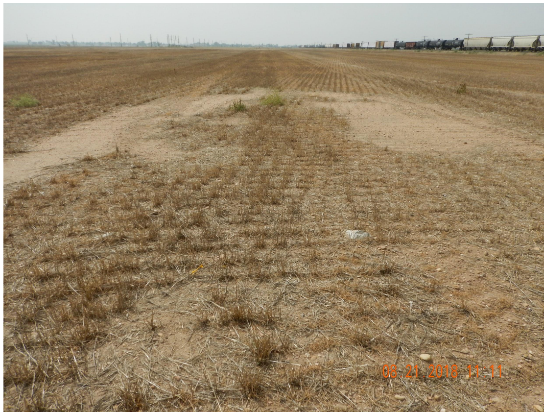
Photo 1. Photo taken from the well location, facing South. Operator has failed to perform all final reclamation activities. There appears to be some gravel and decompaction has not been performed. Last years crop was not able to establish due to the above failed conditions.
