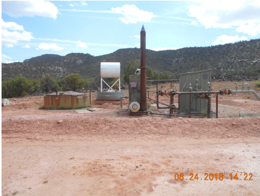
Separator, Meter housing and blowdown tank
