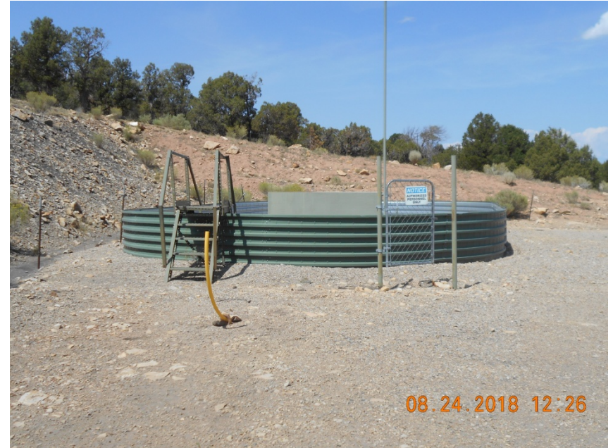
Tank in metal berms. Marked anchor.
