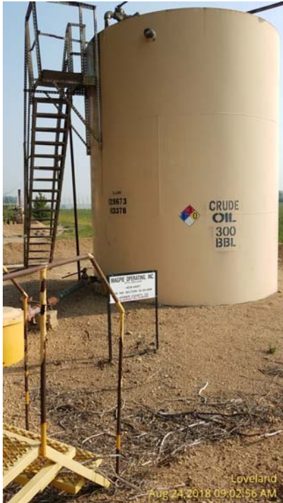
Photo 1 – Sign and crude oil AST at tank battery.
