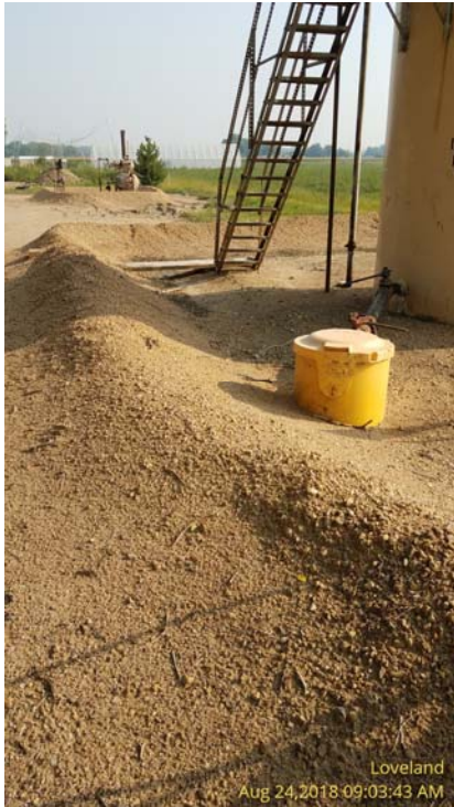
Photo 3 – Containment berm wearing at loadout at crude oil AST.
