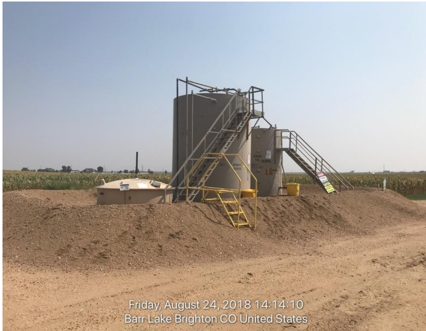
Photo#1 Production Tanks and Produced Water Pit
