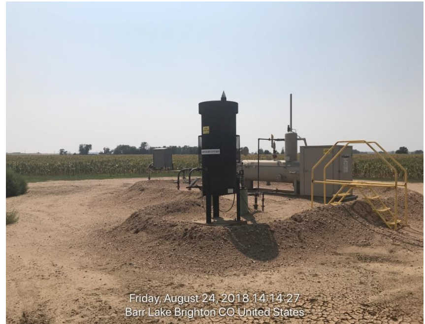
Photo#2 ECD/separator/gas meter
