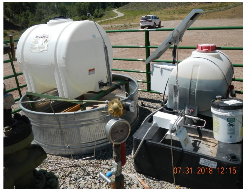
Chemical injection systems in stock panel enclosure adjacent to well head.
