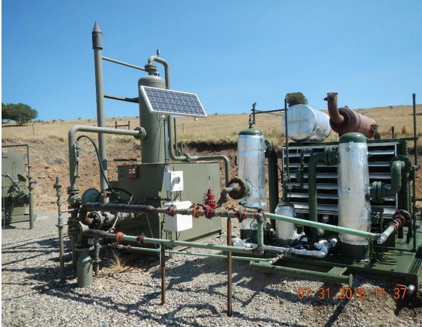
Vertical heated separator and skid mounted compressor.
