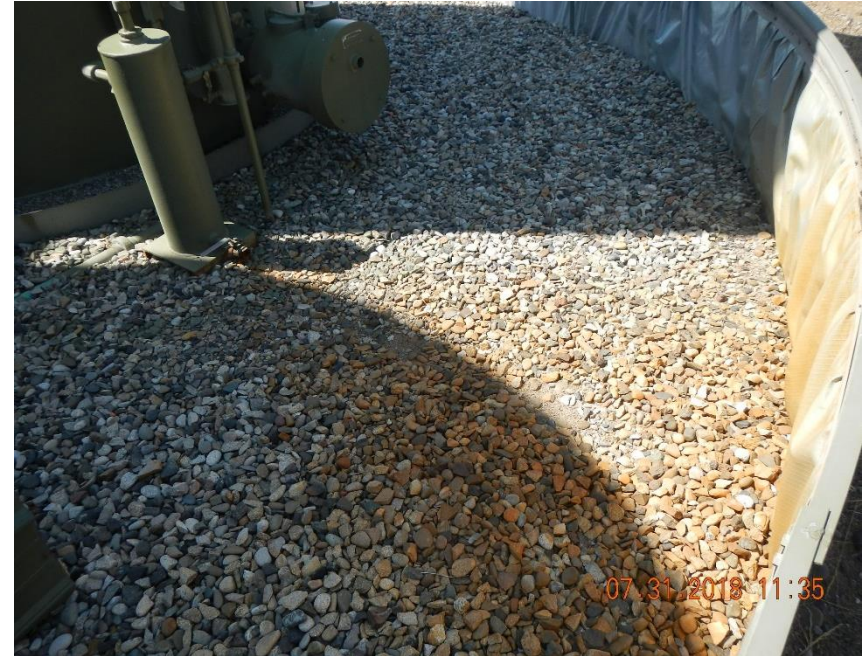
Drop out tanks on tank heaters are being blown down onto gravel.
