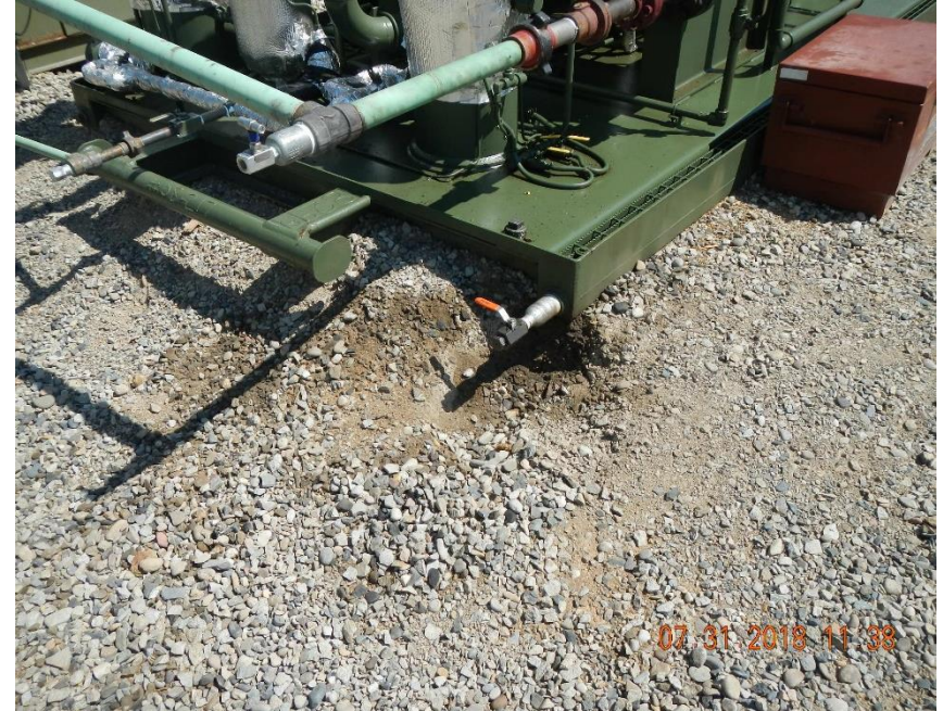
Stained soil around drain outlet for compressor.
