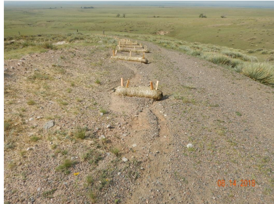
Photo 16: Photo taken from the access road gate, north of the location facing south. Photo shows additional controls have been installed along access road, however, stormwater erosion degradation does not appear to have been repaired, and controls do not appear to be sufficient to mitigate stormwater degradation. See photos 1-4 for additional stormwater concerns on/from access road.
