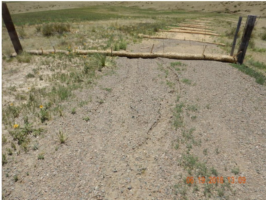
Photo 1: Photo from Inspection #682503518 dated 6/19/2018 (photo #16). Photo taken from the northwest end of the location, facing south. Previous inspection documented erosion degradation along access road and wattle/erosion log no longer in proper functioning condition as stormwater erosion was cutting underneath the wattle. Previous inspections required operator to perform stormwater management
