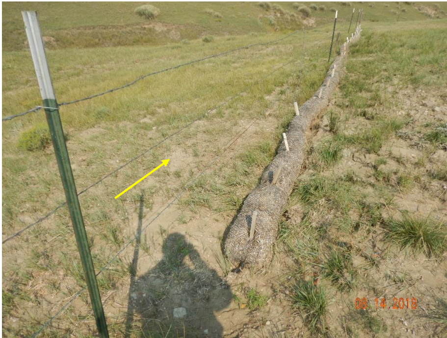
Photo 15: Continued from photo 14. Photo shows sediment from sediment laden stormwater discharge has continued to transport sediment off location..
