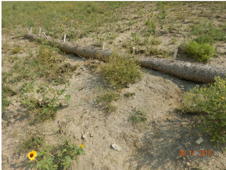
Photo 13: Photo taken from the southern end of the location, facing north. Though some maintenance has been evident on some of the controls on location, sufficient maintenance and stormwater management does not appear to have been conducted or occurring per corrective actions. Photo shows stormwater appear be continuing to cut beneath wattles and erosion degradation has continued on the location.
