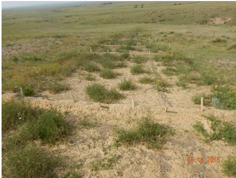
Photo 7: Photo taken from the area of the reclaimed access road on the west end of the location, facing south. Photo shows hydromulching and additional maintenance to properly install stowmater and sediment erosion controls appears to have been conducted.
