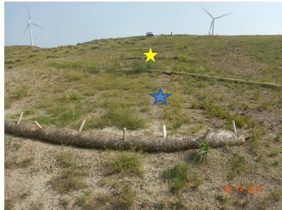
Photo 8: Photo taken from the area of the reclaimed access road on the west end of the location, where access road ended and began traveling east to the well. Photo facing north. Photo shows areas of the access road where gravel/road base has not been removed. Blue and yellow stars show areas where photos 9 and 10 was taken.
