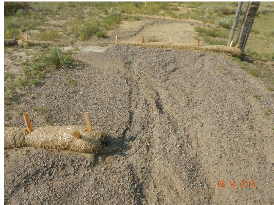
Photo 2: Photo date 8/14/2018. Photo taken from the northwest end of the location, facing south. Photo shows wattle appears to have been replaced, however, BMP has now filled with sediment and is no longer in proper functioning condition. Additionally, stormwater erosion degradation observed along access road has not been sufficiently repaired or stabilized and has been allow to continue.
