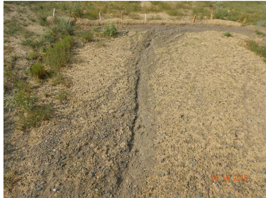
Photo 6: Photo taken from the area of the reclaimed access road on the northwest end of the location, facing south. Photo shows stormwater erosion degradation has continued. Wattle (erosion log) appears to have filled with sediment, and stormwater now appears to be diverting west around the wattle.
