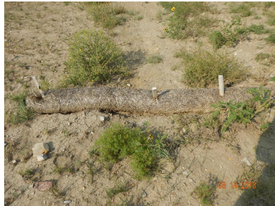
Photo 12: Photo taken from the location. Photo of wattle. Unable to find evidence that maintenance has occurred. Wattle does not appear to have been installed or maintained in accordance to good engineering practices or per corrective actions. Stormwater appears to be traveling under wattle.
