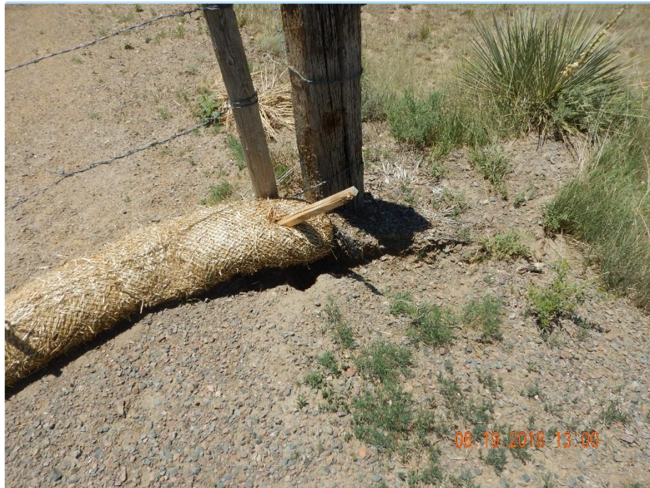
Photo 3: Photo from Inspection #682503518 dated 6/19/2018 (photo #3). Photo taken from the entrance gate of the location. Photo shows stormwater erosion occurring at the entrance with sediment deposition traveling off the location. See comments under photo 1.
