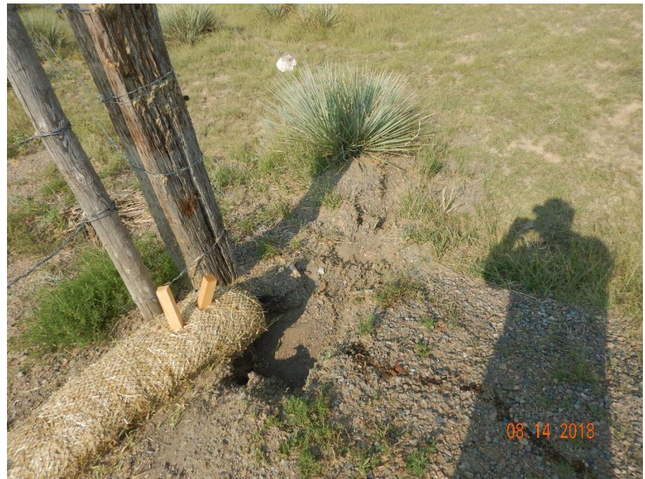
Photo 4: Photo date 8/14/2018. Photo taken from the entrance gate of the location. Photo shows stormwater erosion degradation has not been repaired or stabilized, and degradation and sediment transport off location has been allowed to continue.
