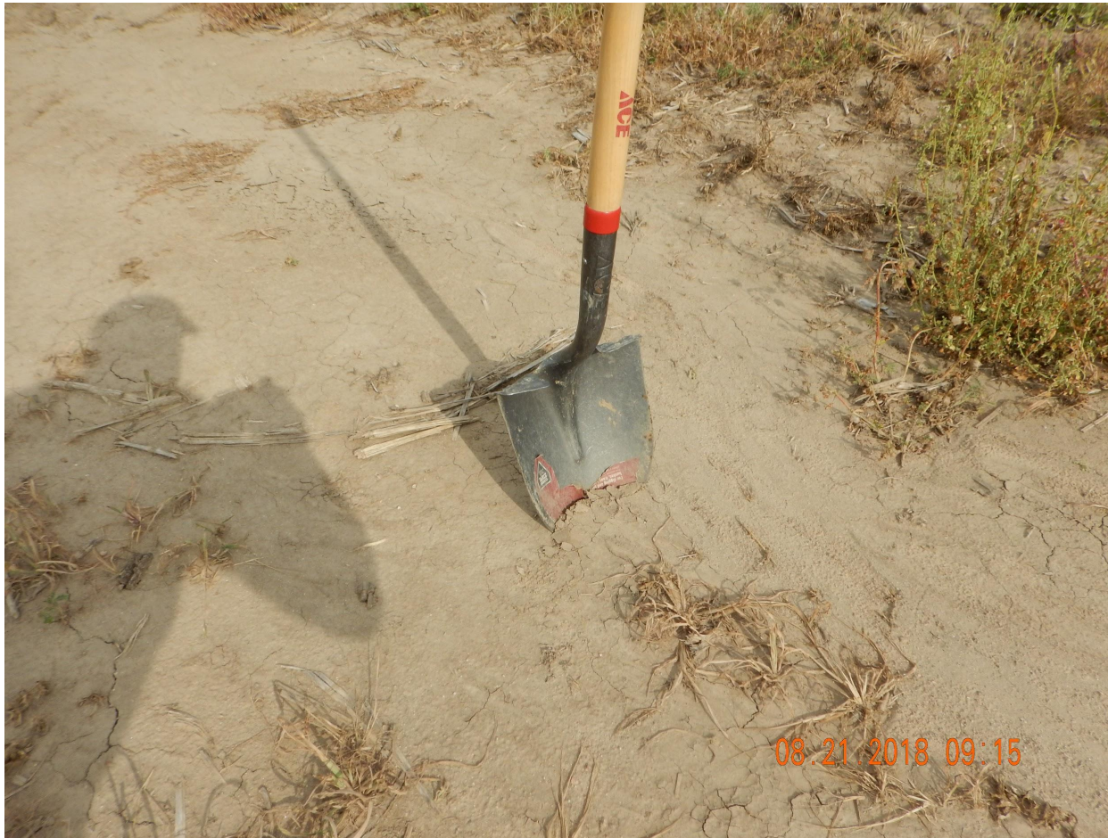
Photo 8. Photo taken from a portion of a compacted area (blue line in first slide) from equipment and vehicle traffic. Operator shall properly decompact to a depth of eighteen (18") inches on all impacted areas. Once the area has been properly decompacted, Operator shall ensure a firm but friable seedbed preparation has been performed.
