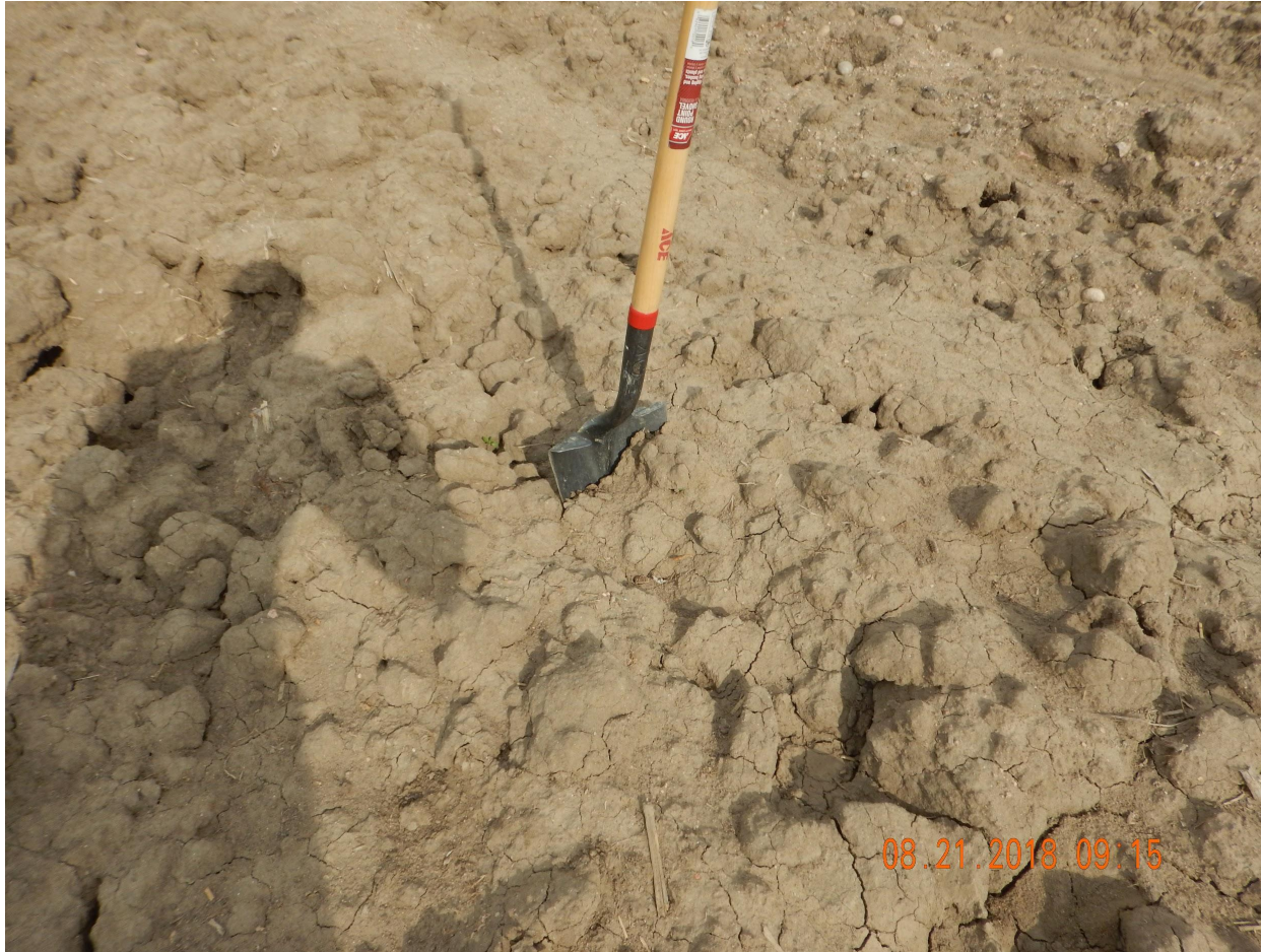
Photo 7. Photo taken from a portion of the excavated area. Photo illustrates excavated areas appear to be decompacted. COGCC Staff did not make an assessment on whether proper decompaction was performed to a depth of eighteen (18") inches per Reclamation rules. Operator shall properly decompact to a depth of eighteen (18") inches on all impacted areas.
