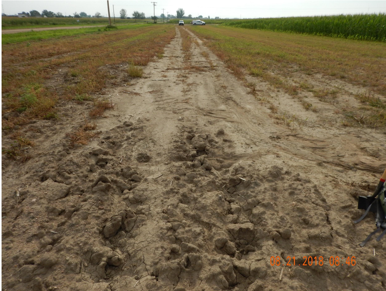
Photo 9. Photo taken from the eastern spill/release point, facing East. Photo illustrates the ~400' area of compaction. Operator shall properly decompact to a depth of eighteen (18") inches all areas impacted areas. Once the area has been properly decompacted, Operator shall ensure a firm but friable seedbed preparation has been performed.
