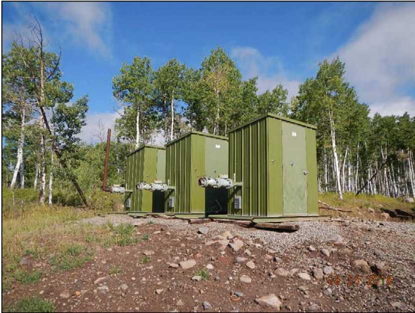
Photo 3. Disconnected separators.
